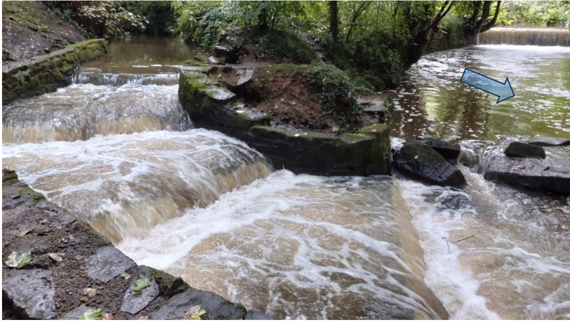
Fig 4. The four steps of the fish pass at the d/s end of the goit where it enters the Yarrow. There appeared to be a series of slightly offset notches to focus flow between the steps under lower flow conditions. NB the diversion of flow from RB to LB u/s of the fish pass on the Yarrow (blue arrow).
