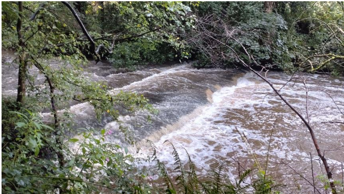
Fig 8. SD 54619 17993: three-tiered step weir looked to be degrading at ~75% of the width from the RB which may be improving the situation for fish passage – see Fig 9.
