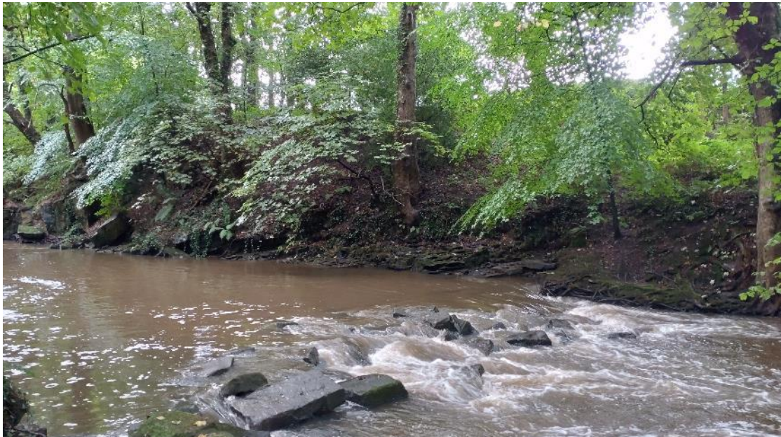
Fig 5. Looking across the Yarrow from RB to LB (from the fish pass; Fig 4) at the redirection of focal flow. This could potentially be more attractive to fish moving u/s, drawing them to the weir rather than the fish pass mouth.
