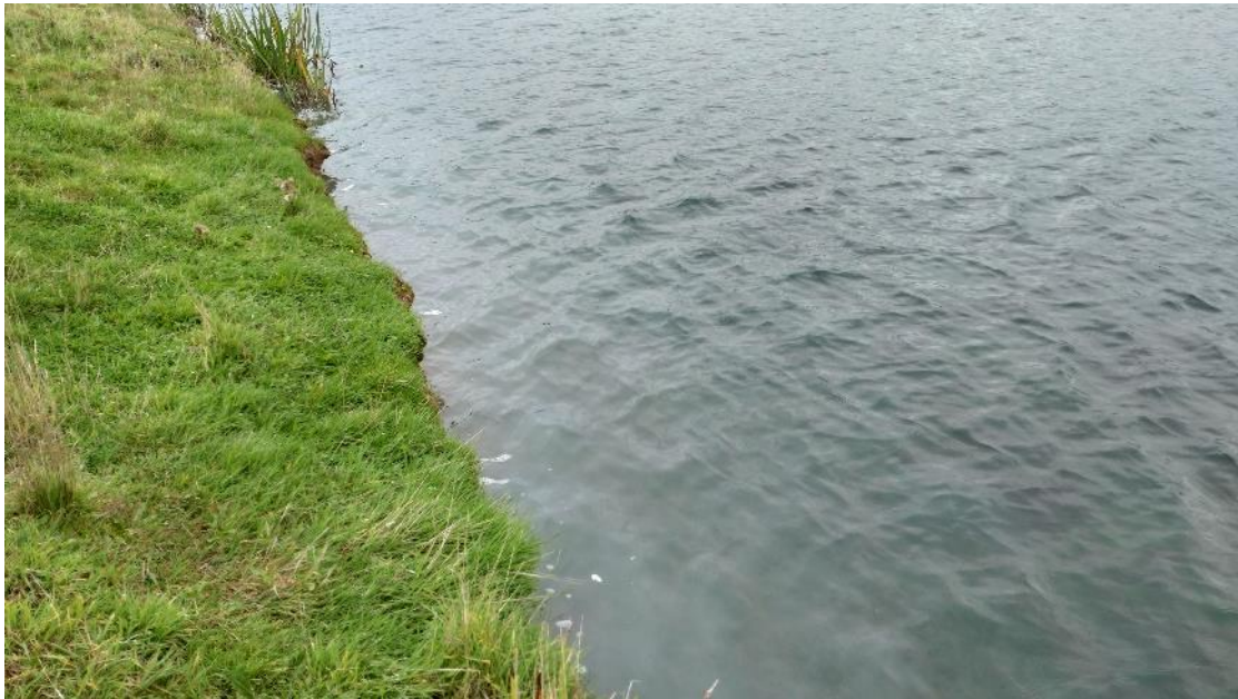
Fig 21. Close up of modest wind action and fetch, yet there was evidence of turbidity from bank erosion along the shoreline. Note that keeping the grass mown as a short sward will exacerbate this problem, as well as make it more attractive for grazing / roosting waterfowl.
