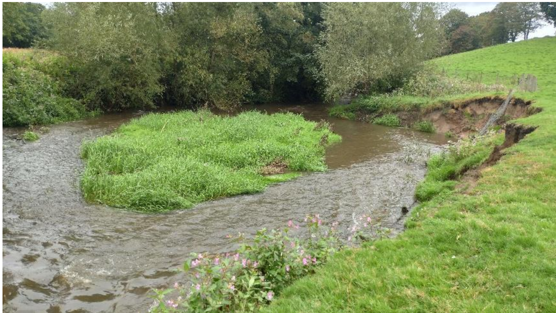
Fig 14. SD 54017 17975: Channel diversification providing different habitat types within the two channels around the island. Unfortunately, the riparian buffer fencing had been placed too close to the bank top again and so had failed, exacerbating the potential for erosion into the RB.
