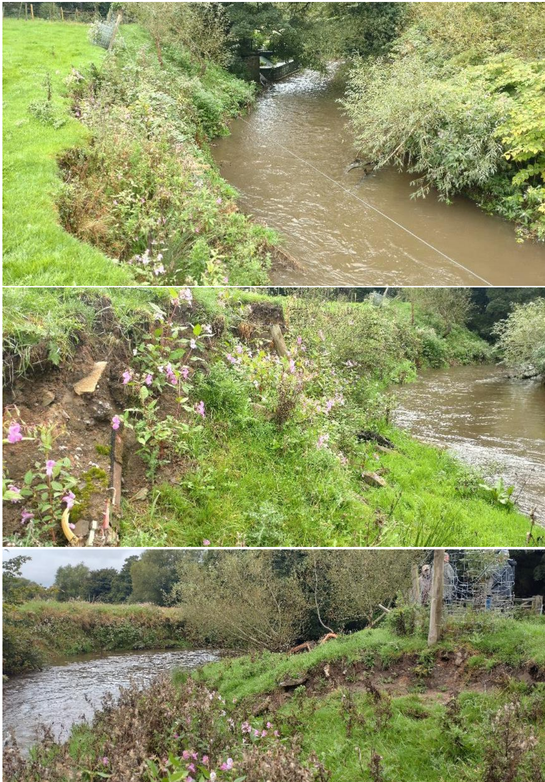
Fig 13. At SD 54184 17978, d/s from the footbridge, the RB had been historically raised to form flatter agricultural land but the fencing protecting the bank had been placed too close to the bank top and deliberately removed in places, thereby allowing stock access. A combination of artificial, unconsolidated bank material (building rubble, metalwork etc, evident in middle image), stock access and Himalayan balsam, with a naturally friable sandy soil anyway, rendered the banks susceptible to erosion by both the water and by stock. Note the large stand of Japanese knotweed on the LB that had not been treated (upper panel).
