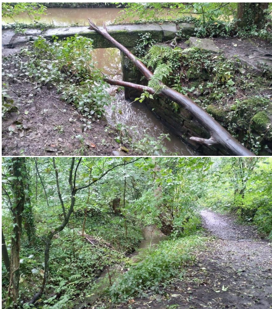
Fig 1. At SD 54790 18010, the u/s extent of the waters and the walkover, the goit associated with the weir was routed from the RB in a heavily incised channel of consistent proportions. Re-naturalisation of the riparian flora had resulted in a native woodland canopy of mixed age, although ground cover was limited due to a relatively dense canopy and the proximity of a popular footpath adjacent.
