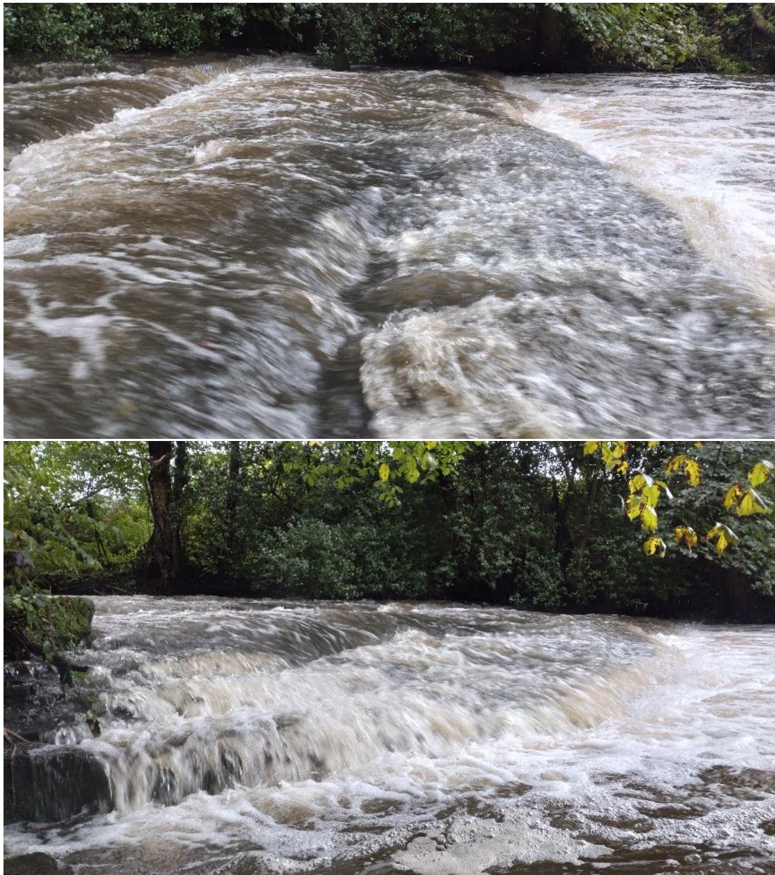
Fig 9. Closer detail of the structure of the weir – broad steps of \sim 1\text{m} base and each \sim 0.3\text{m} high to give a total head loss across the structure of \sim 1\text{m} . Impassable to most fish species the majority of the time. Passability is probably further reduced under lower flow regimes as each step will only be covered by a shallow skim of fluming flow.
