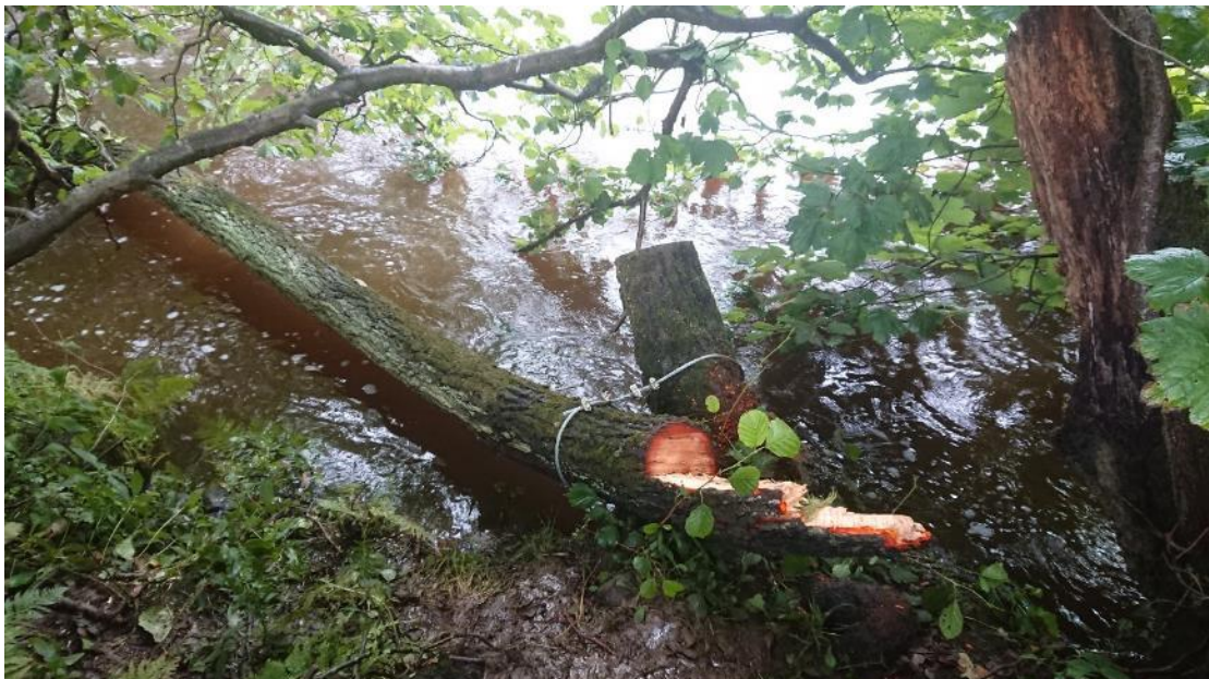
Fig A3. Alder of ~350mm girth felled and cabled back to the living stump as a tree-kicker. The coppiced stump will regrow vigorously, providing further low cover and screening of the cable.
