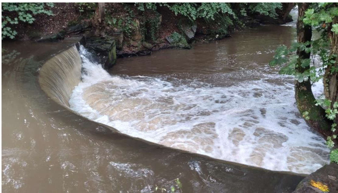
Fig 2. The 1m high, vertical weir had been sited on a seam of bedrock visible on the left bank and was causing impoundment for \sim 150\text{m} u/s. The structure was concave, focussing flow with a slight bias initially to the RB, and clearly an impassable barrier to most fish species most of the time.
