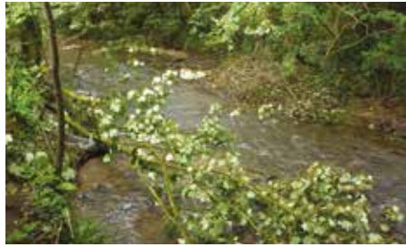
Above: Two of the tree kickers which we've installed in the River Frome in Rodden Meadow
