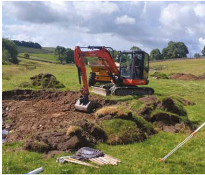
Left: Bank lowering and lateral connection on Flasby Beck at Hetton. Right: The artificially straightened channel of Flasby Beck to the left and a full paleochannel reconnection to the right, to divide the flow energy and allow to develop naturally over time
