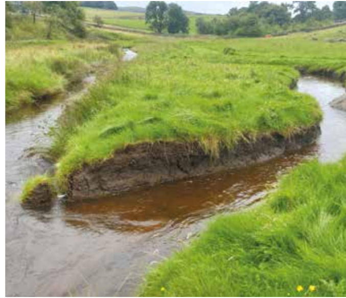
Left: Bank lowering and lateral connection on Flasby Beck at Hetton. Right: The artificially straightened channel of Flasby Beck to the left and a full paleochannel reconnection to the right, to divide the flow energy and allow to develop naturally over time
