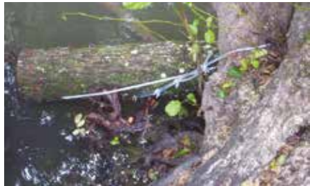
Below: Each tree kicker is secured back to its stump with a short length of steel cable
