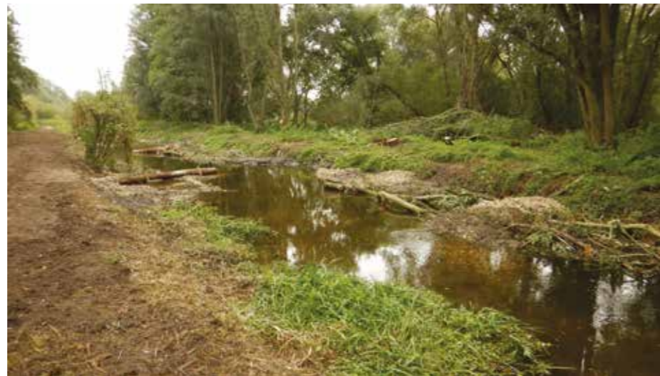
Above: The previously over-wide River Lark at West Stow in Suffolk with no flow diversity to transport fine sediment. Below: The Lark following the creation of log berms backfilled with gravel in September 2022
