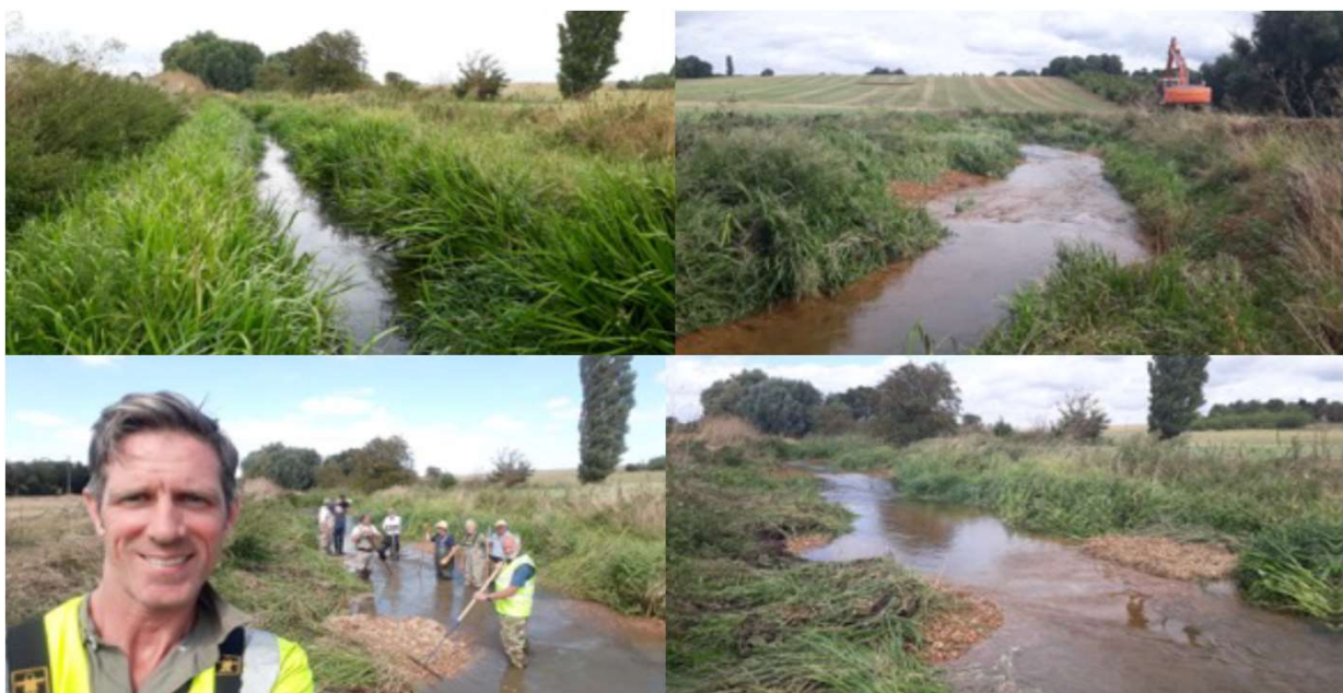
Figure 3a: the River Gwash: top left, a reed-filled stream and clockwise, machines and people open it up, add gravel and produce a more functional river. Note the landmark tree top right of three photos.
