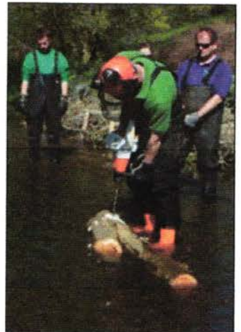
River Forth Fisheries Trust put WTT advice into practice in the Allan Water, Central Scotland to repair an eroded bank and create great habitat along the river margin (photo: River Forth Fisheries Trust)
