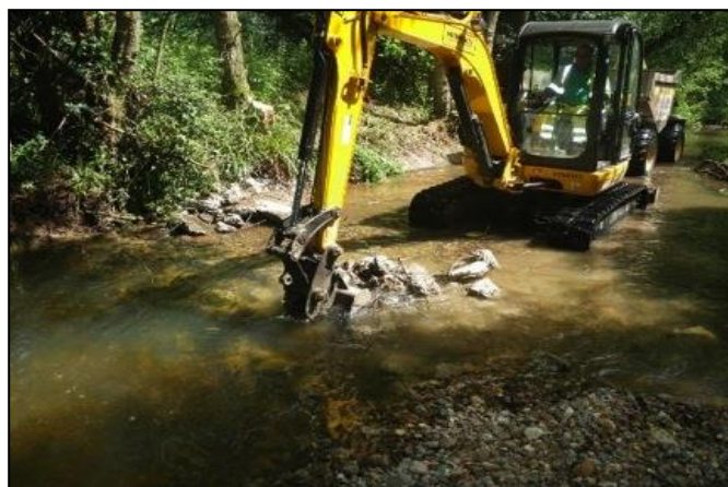
Fig. 5a: The Monks Brook, in its concrete jacket (left). Works starts, digging into the concrete, then...
