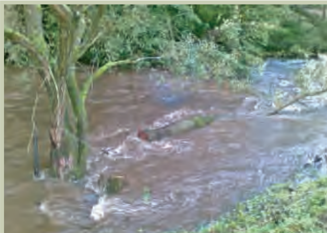
LWD CABLED TO LIVING TREE PICTURED DURING FALLING SPATE FLOWS ON DERBYSHIRE'S RIVER GOYT...
