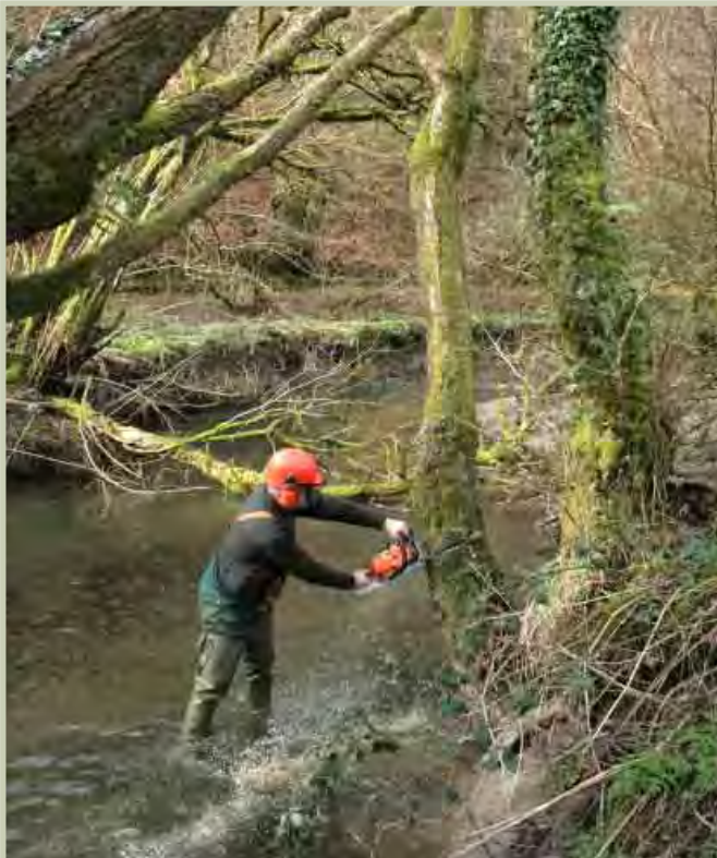
'HINGING' LWD FOR INTRODUCTION INTO AN UPLAND STREAM
