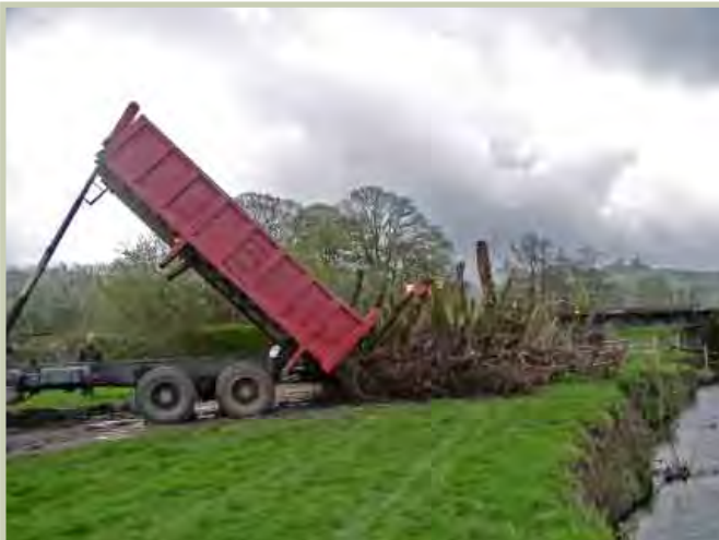
ROOT WADS DELIVERED TO SITE.....
