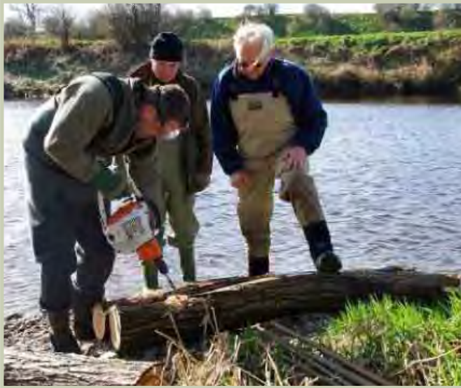
DRILLING LARGE WOODY DEBRIS PRIOR TO INSERTING REBAR
