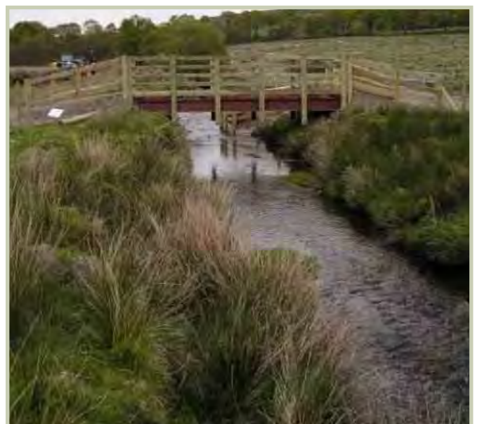
A WELL SITED STOCK ACCESS BRIDGE
