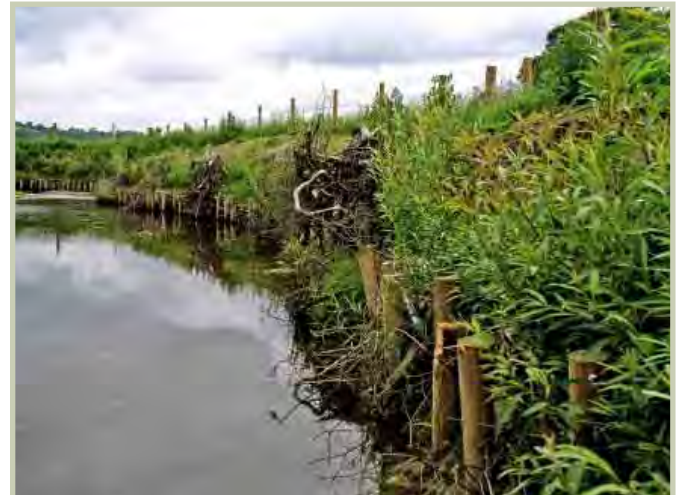
.. AND INSTALLED WITH LIVE WILLOW TO PROTECT BANK
