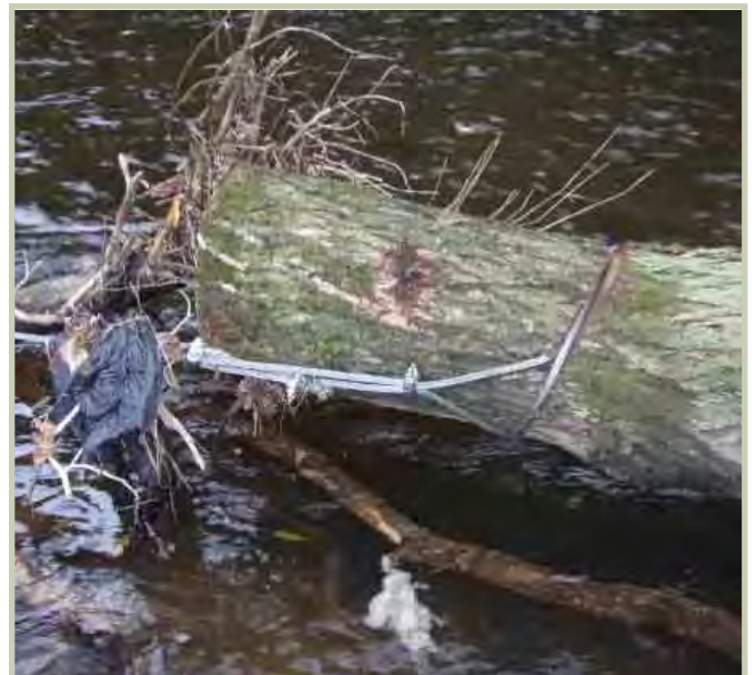
DETAIL OF WIRE RETENTION SYSTEM FOR LWD
