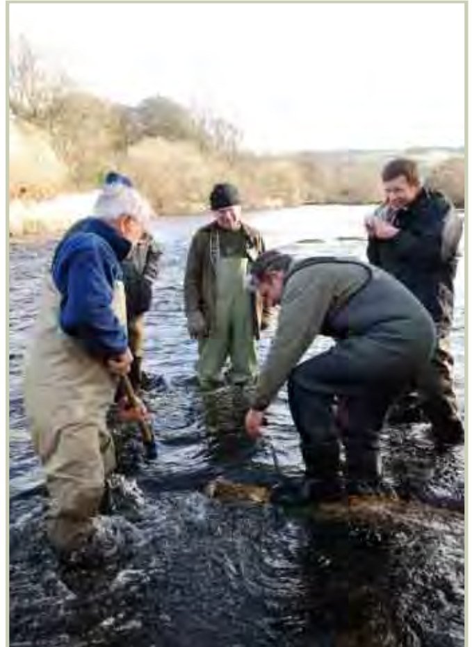
USING REBAR TO FIX LWD IN THE CHANNEL
