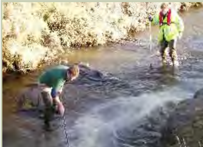
APPLYING LIMESTONE SAND TO A HEADWATER STREAM IN THE TOWY CATCHMENT
