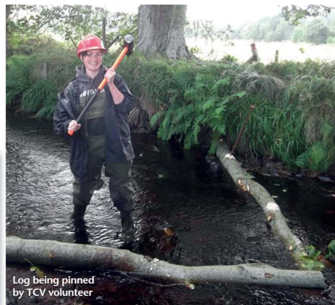
TCV volunteers building the last structure - two log deflectors
