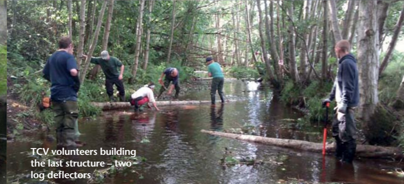
An example of a log deflector on the River Peffery. The log does not always have to go all the way across the channel. The deflectors are kept low so they do not cause impoundment and flood flow can go over them easily
