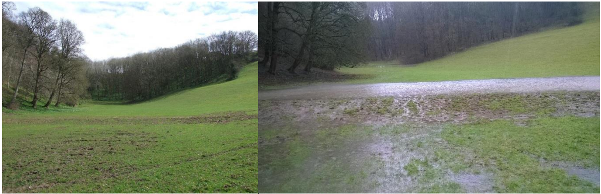
Upper Painswick Valley field bund in normal and flood flow conditions
