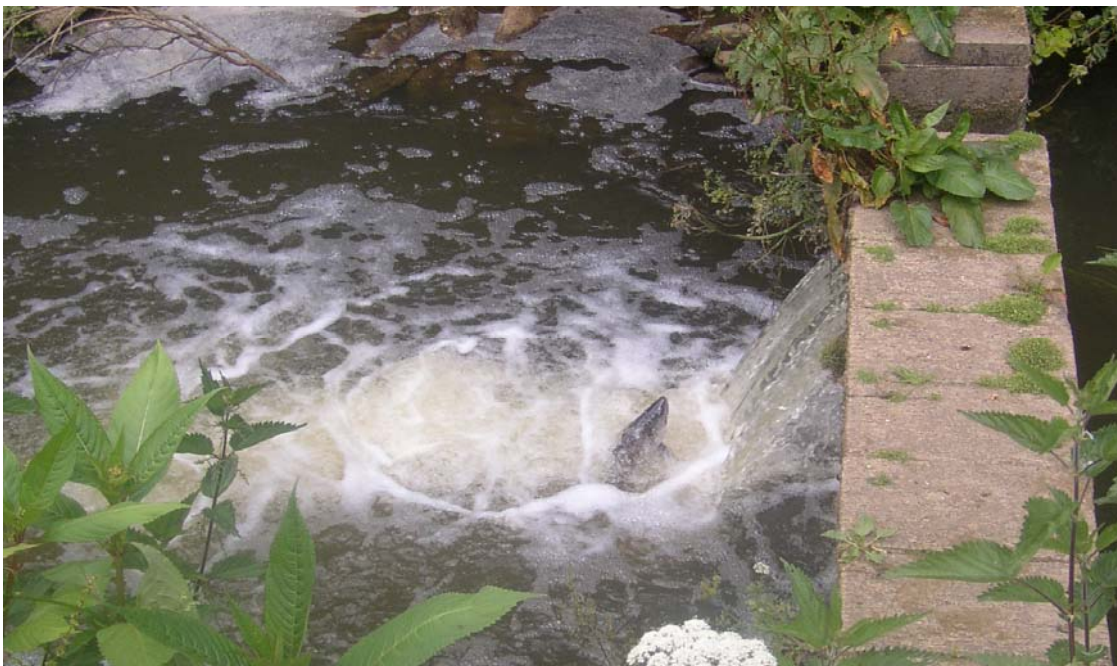
Fig.(17) Obstructions to fish passage at Barcombe on the Ouse
