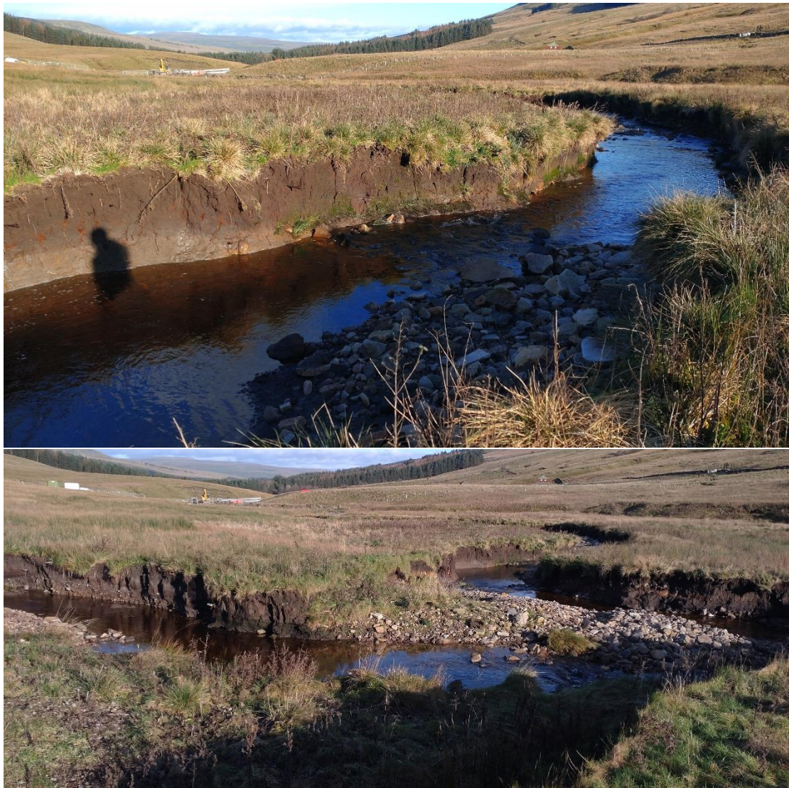
Fig 5. Meanders within the section highlighted from Fig 3. The channel was highly incised, probably resulting in part from the straightening of the channel reaches downstream accelerating flow velocity and increasing erosive power within an area which was clearly more depositional in the past (based upon the fine soils above the coarser alluvium). More frequent and intense rainfall events in recent decades, and historic land management practices of drainage and grazing resulting in a lack of tree cover, will have undoubtedly contributed.
