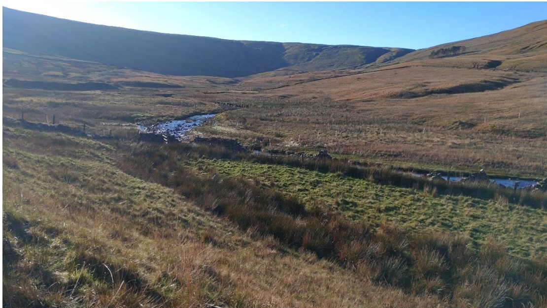
Fig 4. Looking u/s from afar at the low gradient and relatively broad floodplain of the meandering section highlighted in Fig 3.
