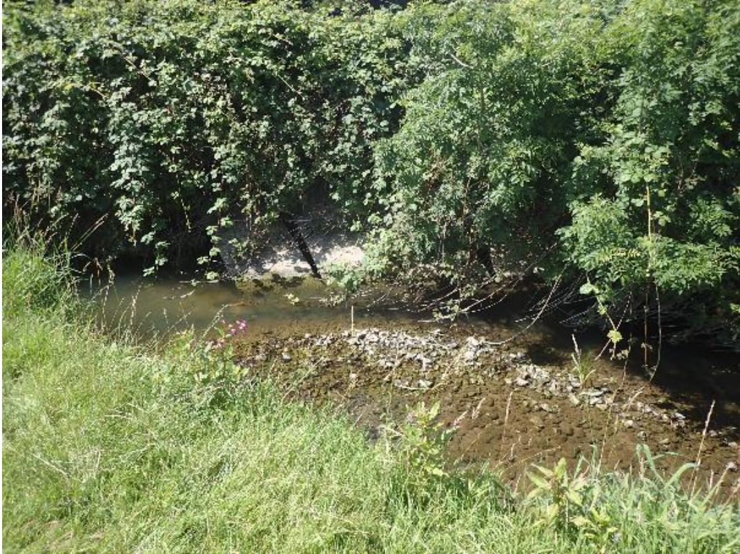
Photo 12: Concrete dumped in the river in the vain attempt to reduce erosion! It simply deflects the river's energy downstream and will eventually fail leaving concrete in the river.
