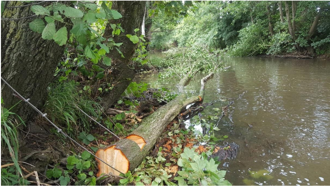
Photo 21: A tree kicker cabled to an existing tree stump on the River Yeo. Kicker tethers should be as short as can be realistically achieved: apart from too much metal cable being unsightly and unnatural, the risks of the trees being stranded on the banks in floods are significantly increased. Hiring or investing in a hand winch would allow the kickers to be winched back toward the stump, reducing the amount of cable needed, which in turn will reduce the likelihood of the kicker being stranded on the bank after high flows.
