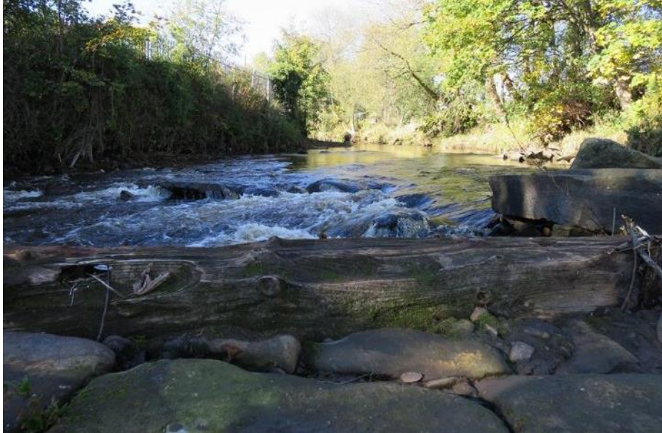
Figure 15: The impounding effect of the weir at SE07216 41705 is reducing as the weir gradually collapses. Habitat in the upstream reach is beginning to improve (note the deposited cobble “point bar” towards the upper, middle part of the frame on the RB).
