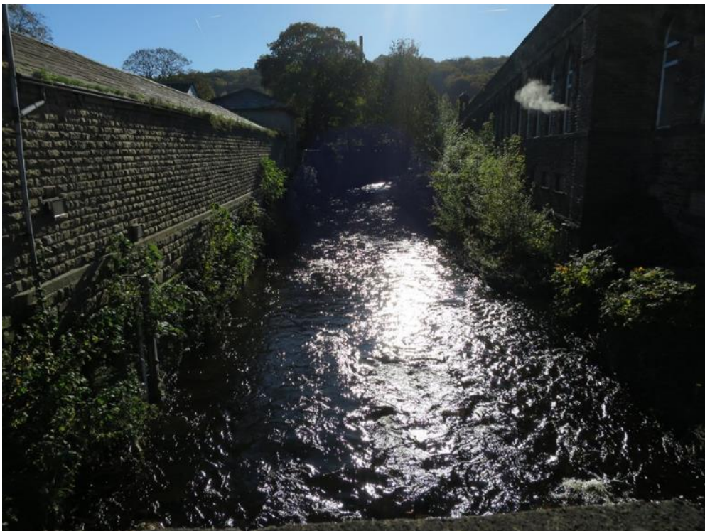
Figure 18: Although facing into the sun, it is possible to see the straightened and constrained character of the river.
