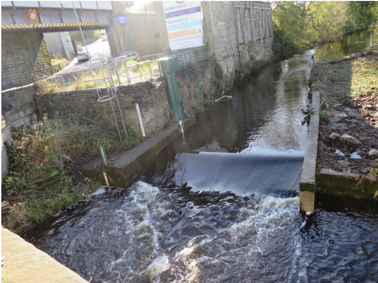
Figure 25: Weir fitted with gauges visible on the RB (left of frame). This installation is probably formally incorporated into EA river levels monitoring. To the right of the frame there appears to be a back-filled lagoon/mill pond which may have been altered to facilitate calibration of flow-gauging. The power of the laminar flow of water over the weir itself is a severe barrier to upstream fish migration.
