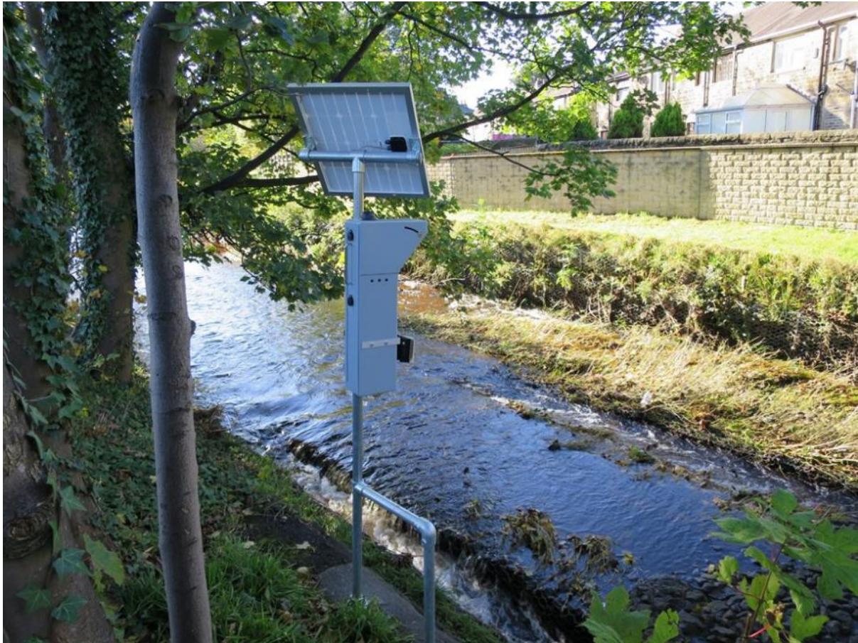
Figure 10: Upstream channel and telemetry/instrumentation associated with the structure.
