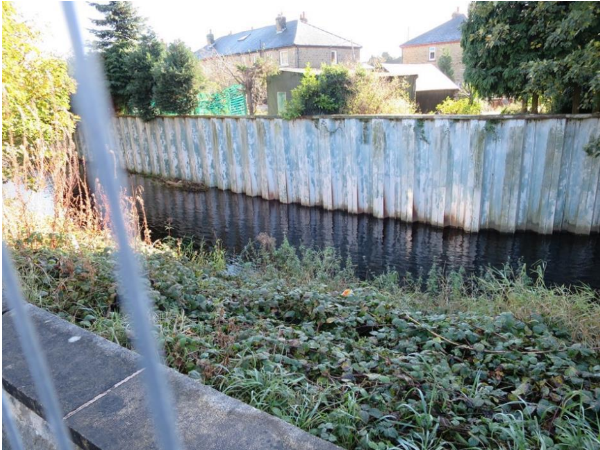
Figure 8: Sheet piling flood defences (showing proximity to housing).
