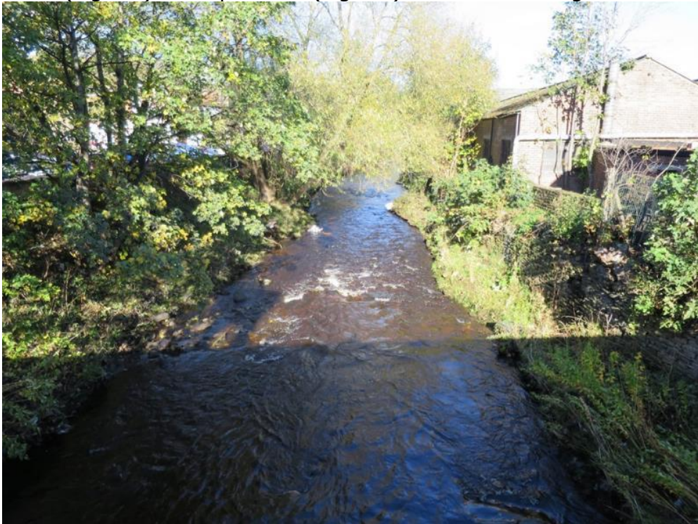
Figure 17: Facing downstream, the high-vertical walls constrain the river to accommodate surrounding development. The high gradient of the river (which is amplified, by straightening since the same vertical change in elevation occurs over a shorter path-length) and development of marginal vegetation help to create slightly more varied habitat than would occur in impounded reaches. The effective increase in gradient by straightening (in an already steep catchment) is one of the factors contributing to the difficulty in managing flood risks at downstream bottlenecks.
