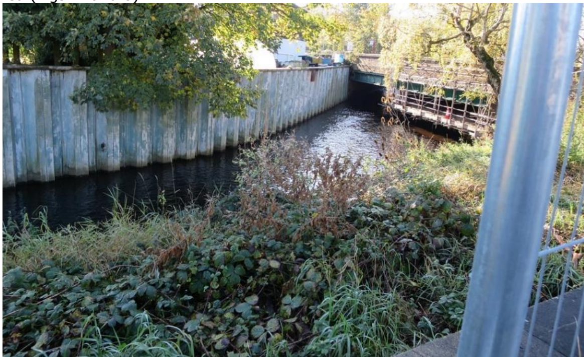
Figure 7: Repair work to bridge and vertical sheet-piling revetments.
