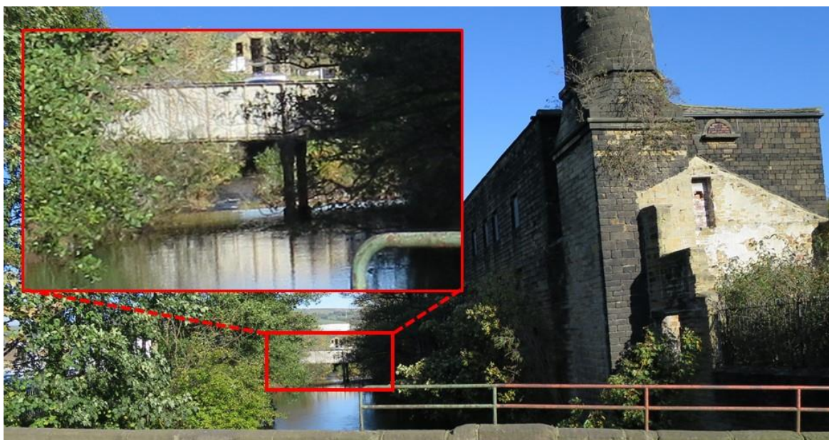
Figure 24: Continuation of impoundment downstream from photograph in Fig. 23. The crest of a large weir is just visible beneath the bridge towards the lower/centre of the frame in the far background (enlarged in the inset). The height-difference between the flat, reflective water at the crest and the more broken water below is substantial.
