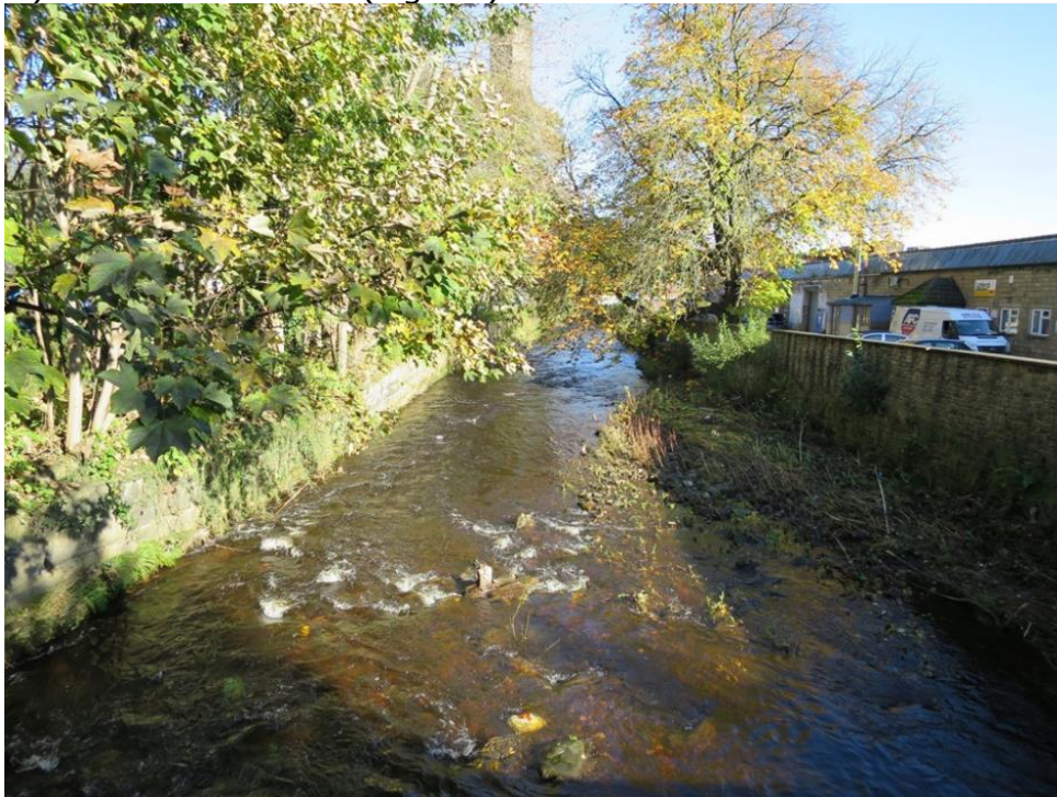
Figure 19: Photo facing downstream at SE 06959 41266. The point bar on the RB (right of frame) is supporting some marginal vegetation growth – which in turn helps to consolidate the depositional feature. This also creates an increase in depth towards the LB (left of frame) by encouraging bed-scour. The result is at least a limited degree of meandering flow within this straightened/walled section of river.
