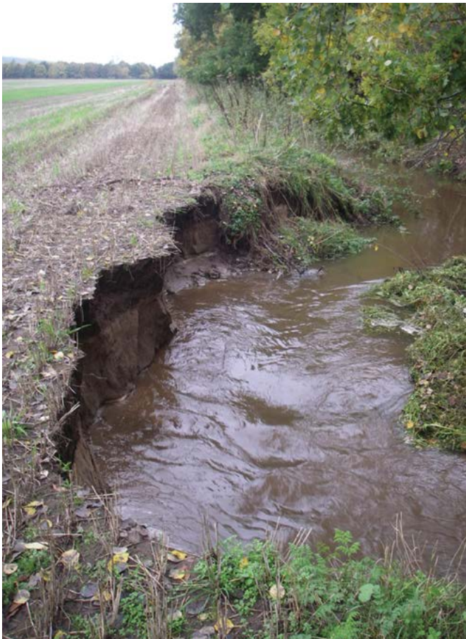
Figure 4.21 The diversion of water around a beaver dam has caused bank erosion at this Tayside site. © Helen Dickinson/TBSG
