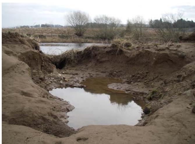
Figure 4.23 Burrowing by beavers led to this breached flood-bank on Tayside. © Helen Dickinson/TBSG
