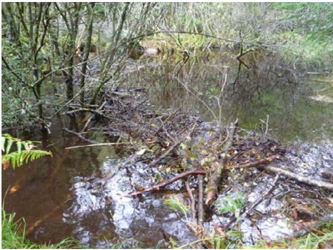
Figure 3.45 Secondary dam on outflow from Loch Linne, Knapdale, September 2009. © University of Stirling (Charles Perfect)/SNH
