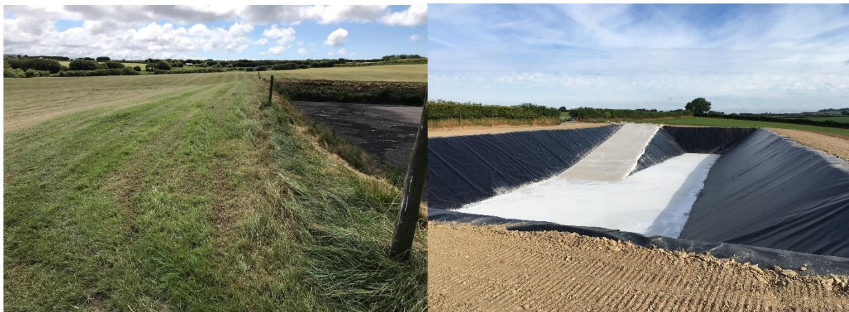
New non-compliant earth bank store
