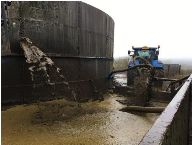
Split in slurry tower
