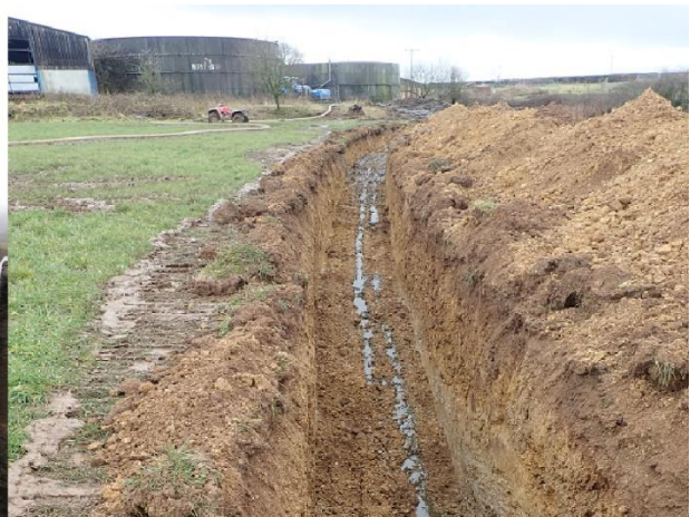
Slurry interception ditch
