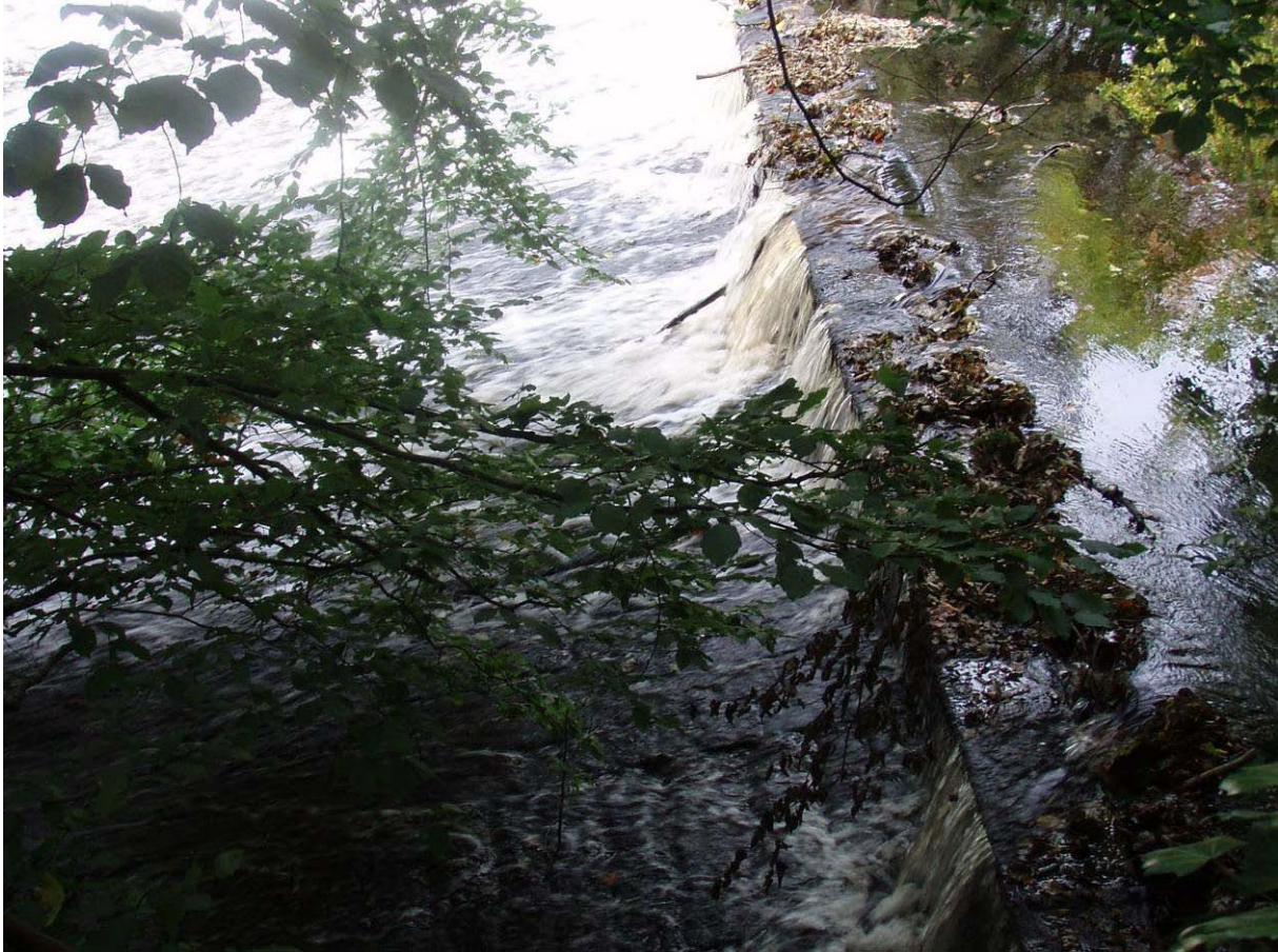
Photo 1 – Weir at the top of Glasshouses mill race. The vertical step at the top makes a difficult weir impassable in all but very high flows. Small fish don't have a chance of ascending it.
