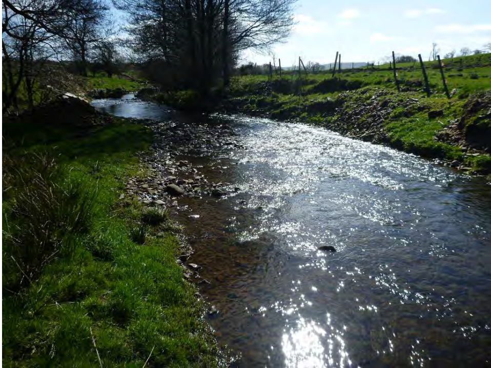
Photo 28 Example of the use of river bed material to shore-up an eroding bank and prevent lateral movement of the river channel. Such activities are damaging to in-stream habitat and prevent the straightened river from re-developing meanders and better trout habitat; if the gravel disturbance is carried out during the fish spawning season (Oct – May), direct damage to fish eggs could be caused. For these reasons, such activities are governed by the Environment Agency’s Environmental Permitting Regulations.
