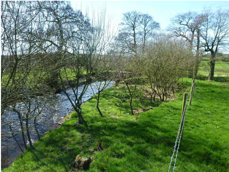
Photo 15 Area indicated by arrow in Photo 14 (downstream view from RHB). Brushwood revetment and willow planting had been carried out here (shown by the line of willows). The area in front of the willows appears to have been filled with river sediments.
