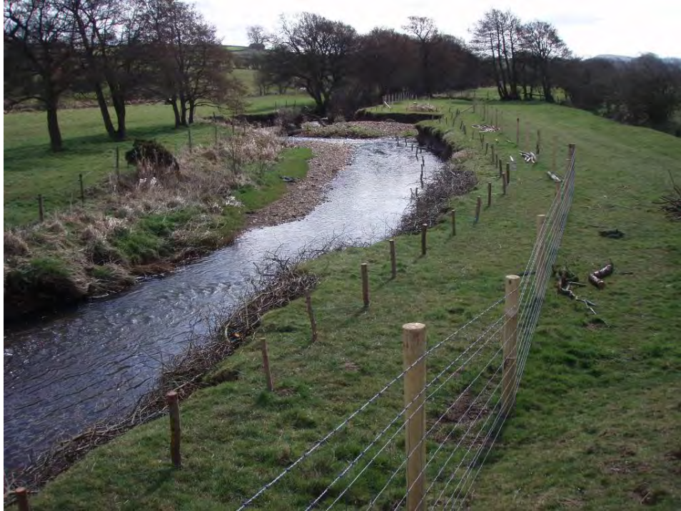
Photo 2 March 2009. View downstream towards the d/s end of the Ludburn beat, shortly after completion of brushwood installation and fencing.
