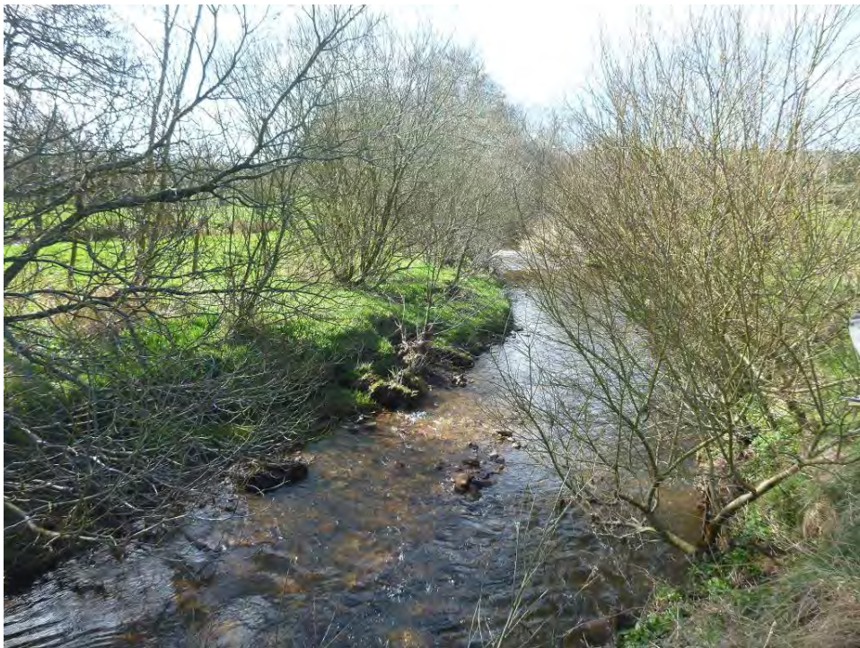
Photo 7 March 2019. The same view as above. The combination of brushwood bank protection and exclusion of livestock (fencing) has been successful, allowing planted willow cuttings to establish, stabilising the bank. The willows on the right bank should be laid over into the water (like hedge-laying). A living willow stake could be driven into the bank to hold the top ends down.
