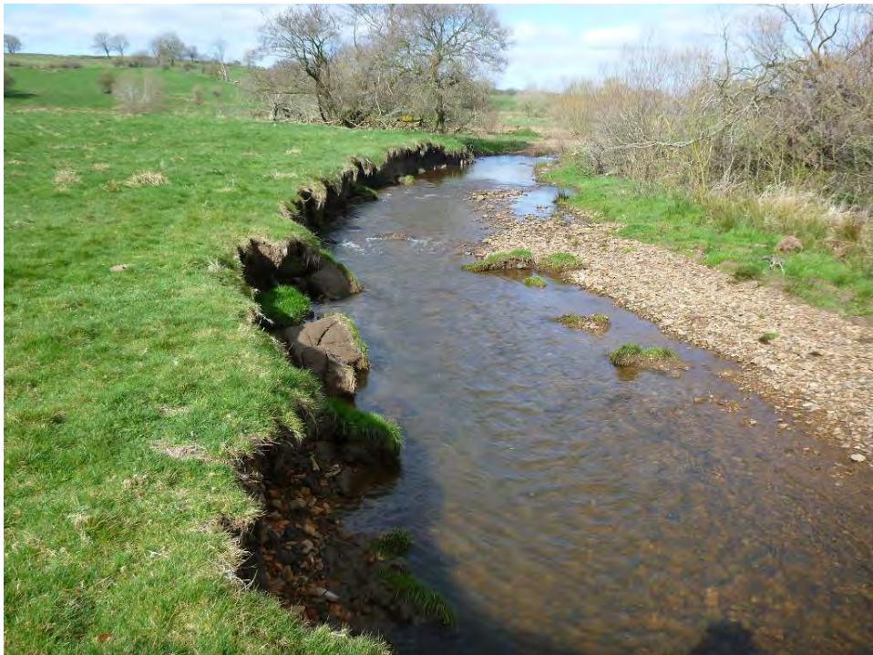
Photo 19 Block failure erosion. Revetment with willow bundles may slow down erosion on sections like this and provide some fish cover, but livestock exclusion would also be required on low banks like this.
