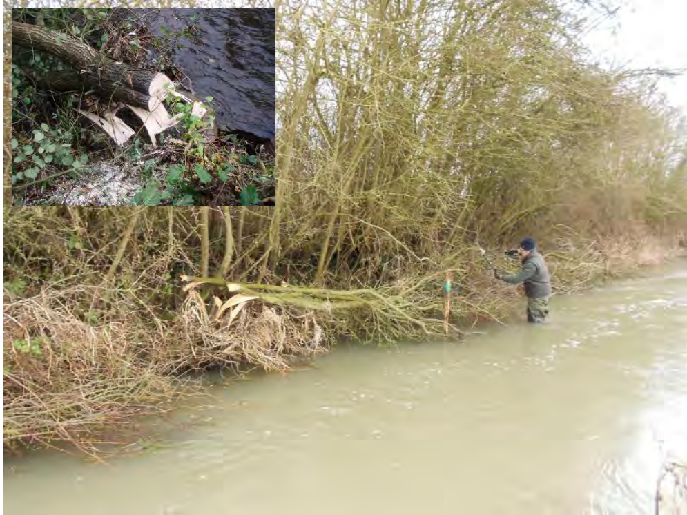
Photo 30 Laying trees into the water to provide excellent cover for trout. Inset: detail of partial cut to retain the tree and keep it alive.
