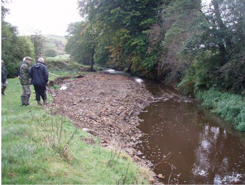
Photo 1 October 2007. Example of unconsented channel straightening and gravel dredging downstream of Windy Arbour Bridge. This prevents the straightened channel from re-gaining sinuosity and better habitat.
