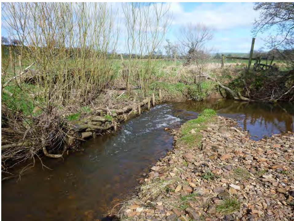
Photo 13 Immediately u/s of Photo 12. Bank protection with woody material and living willow in-fill has successfully protected the bank. The sprouted willow could be coppiced and used to reinforce this area and elsewhere.
