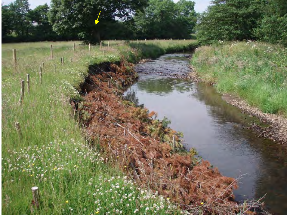
Photo 4 June 2009. First summer after brushwood installation and fencing. Site in first field downstream of Ludburn footbridge (Grid ref of tree indicated by arrow: SK0942962357)
