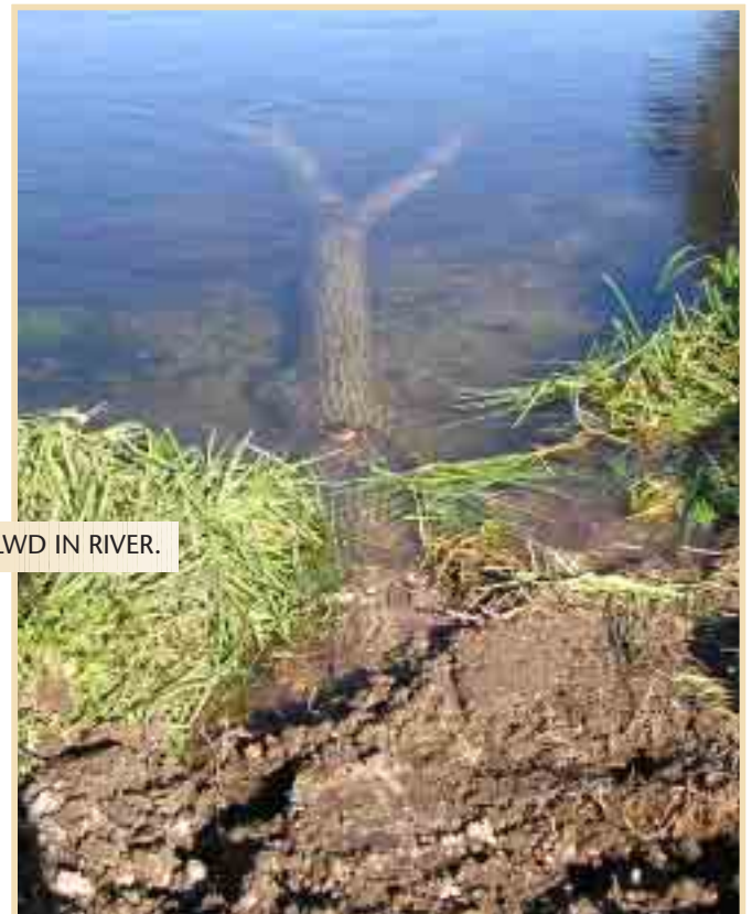
LWD BEING PUT INTO POSITION.
