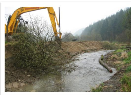
Figure 18. A. Clywedog 2009: Repair in progress
