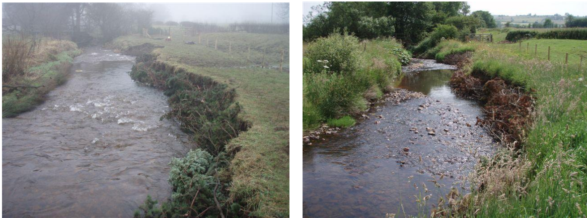
Figure 2: Brush installation (left) and riparian vegetation re-establishment through grazing exclusion (right) creating ideal habitat for juvenile trout
