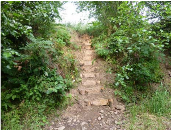
New access steps
