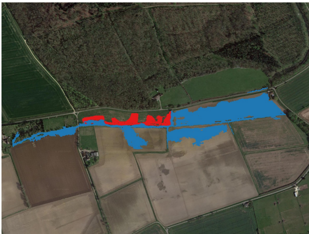
Figure 4.7a 1 in 5yr flood extent change, blue = baseline, red = restored (where red is visible indicates flood extent increase).
