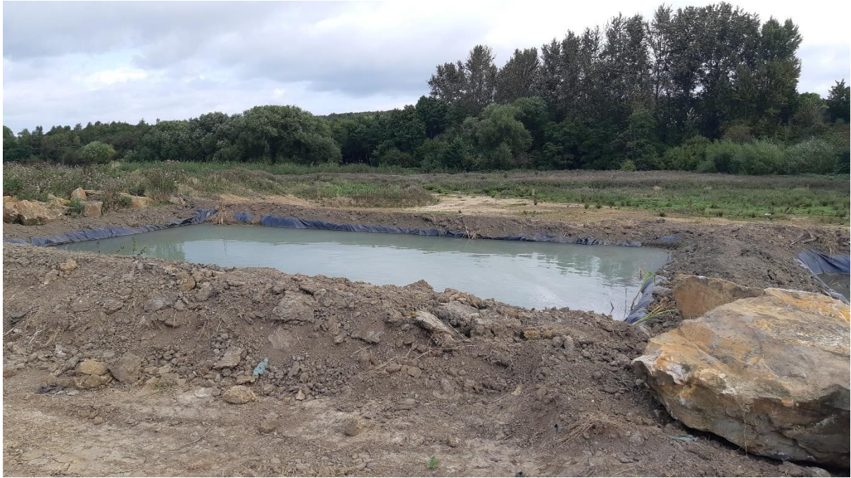
Figure 4: With the river at the foot of the distant treeline, these plastic-lined ponds and (beyond) floodplain vegetation re-establishment may offer a degree of sediment interception. Note the uniformly steep, smooth sides of the ponds are likely to limit their habitat value.
