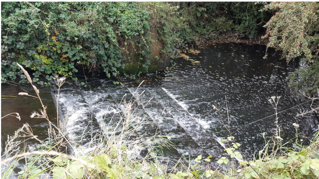
Figure 1: Stepped weir causing both a barrier to migration and inhibition of bed material transport at 53.234167, -1.3125000.
