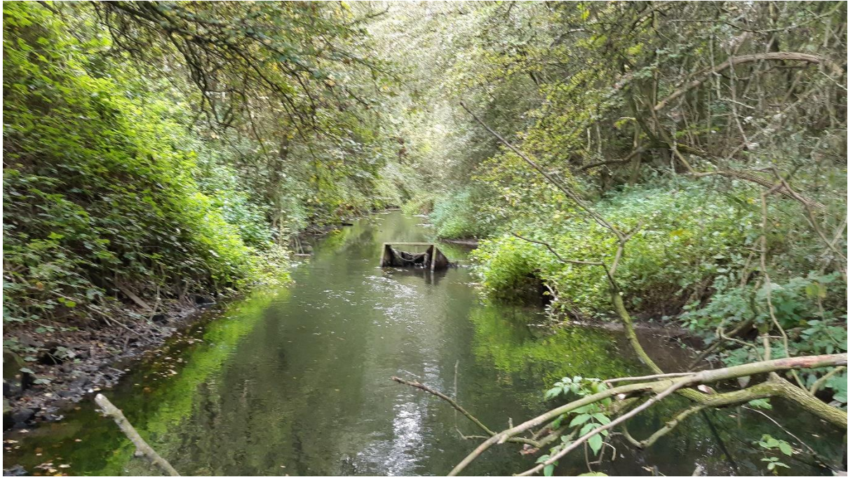
Figure 8: Although flanked by vegetation in this particular reach - the straight "box-shaped" armoured channel generally provides poor habitat.
