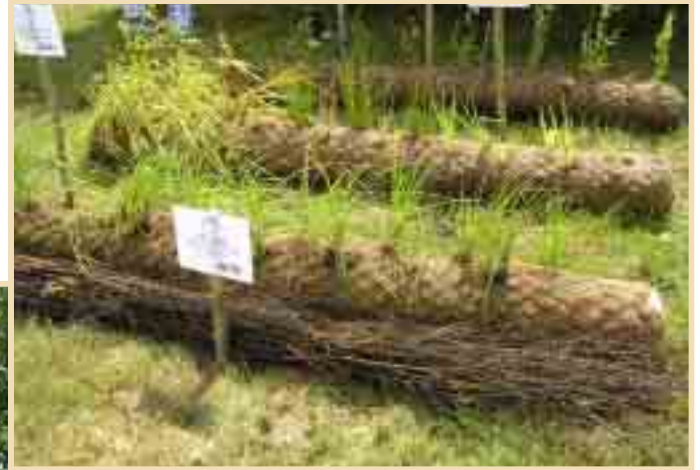
NEWLY-NARROWED CHANNEL USING PREPLANTED COIR FIBRE ROLLS .
