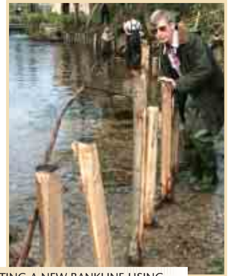
CREATING A NEW BANKLINE USING FAGGOTS AND UNTREATED STAKES.
