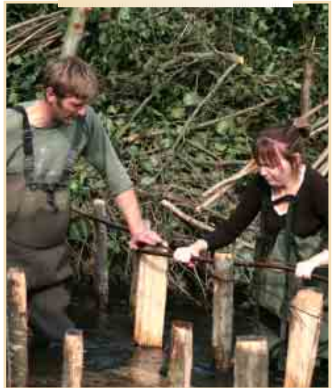
CREATING A NEW BANKLINE USING FAGGOTS AND UNTREATED STAKES.
