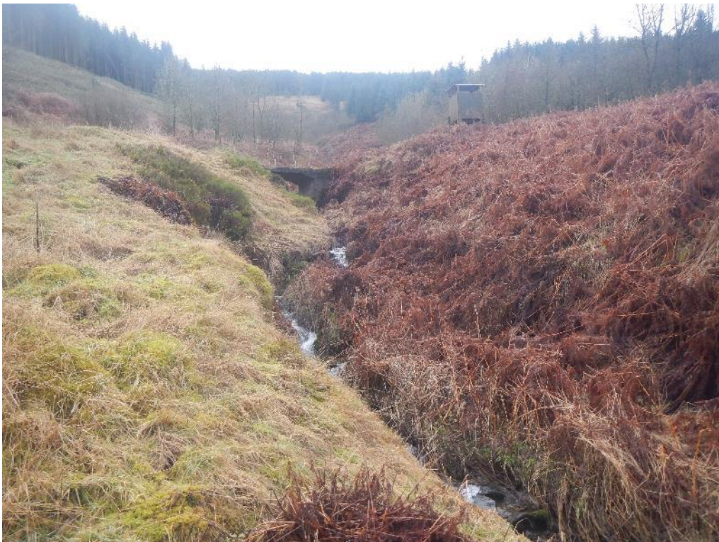
Figure 16. Clackanna Sike is a steep and poorly accessible tributary, with the track crossing creating an additional obstruction (55.1833578, -3.1258847).
