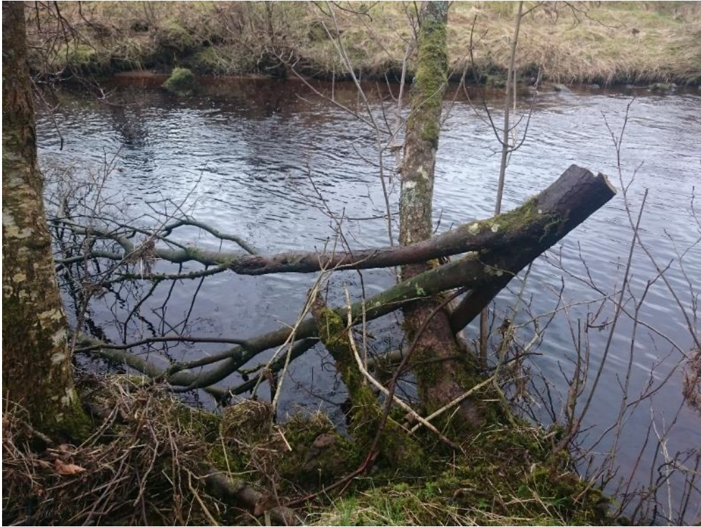
Figure 48. Another variation of lodged woody material, or hanger. This technique is equally secure as the standard lodged woody material. A hybrid of the two techniques can also be applied – demonstrated here during a previous habitat workshop on the River Esk catchment.
