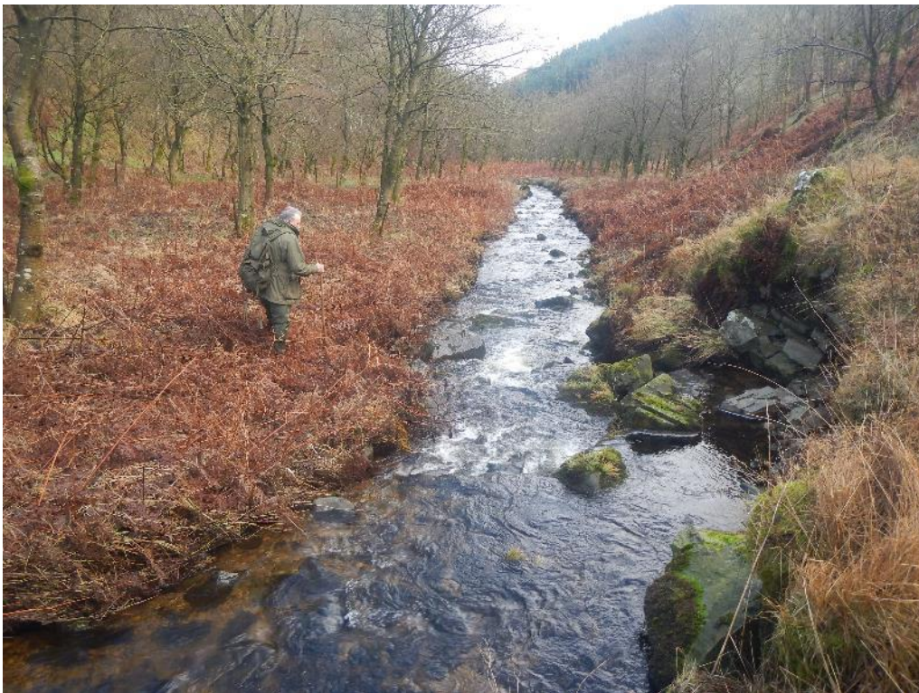
Figure 20. Another straightened section: note the boulder/cobble nature of the straightened, steepened channel (55.185008, -3.119887). The watercourse should be flowing off to the left of shot, as per the previous straightening. Potential for bed raising/restoration to reinstate the paleochannel.
