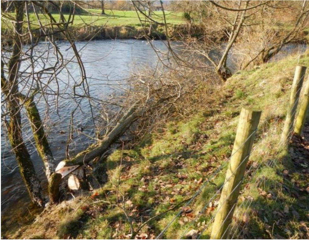
Figure 51. Willow hinged into the river margin to increase cover and structure. The method involves cutting part way through the stem, quickly through the first two thirds, then continuing until it collapses or can be pushed down over the river. The depth of the cut should be limited to only that which is required to bend the stem over, as this will maintain maximum size and strength of the hinge and the health of the tree/shrub.
