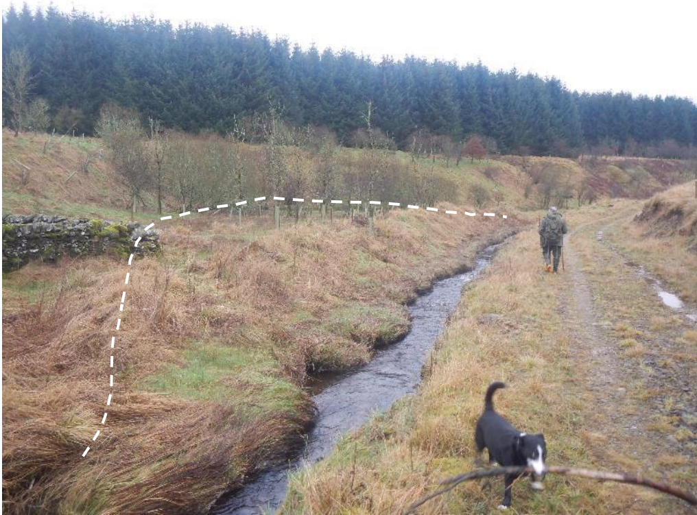
Figure 11. D/s of Trough Burn the now much larger watercourse was also clearly straightened (approximate past course - dashed white line), reducing gravel retention and increasing incision. This channel could be restored (55.18405,-3.132652).
