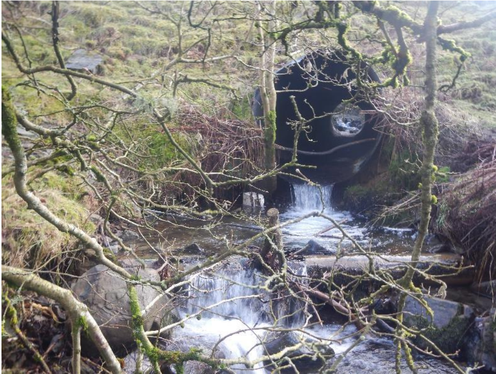
Figure 41. Glenbertle Burn suffers the same issue as many of the southern Boyken Burn tributaries, with fish passage greatly inhibited by a perched track culvert (55.185678, -3.077052).
