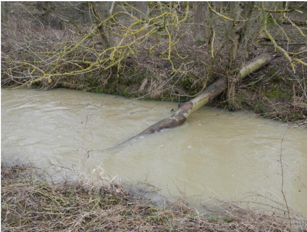
Figure 47. Lodged woody material flow deflector. Note how the two upright sycamore stems lock the pole in place. The more pressure that is exerted by flow, the greater the friction becomes. This cannot wash out unless the well-rooted supporting trees give way, which is highly unlikely.
