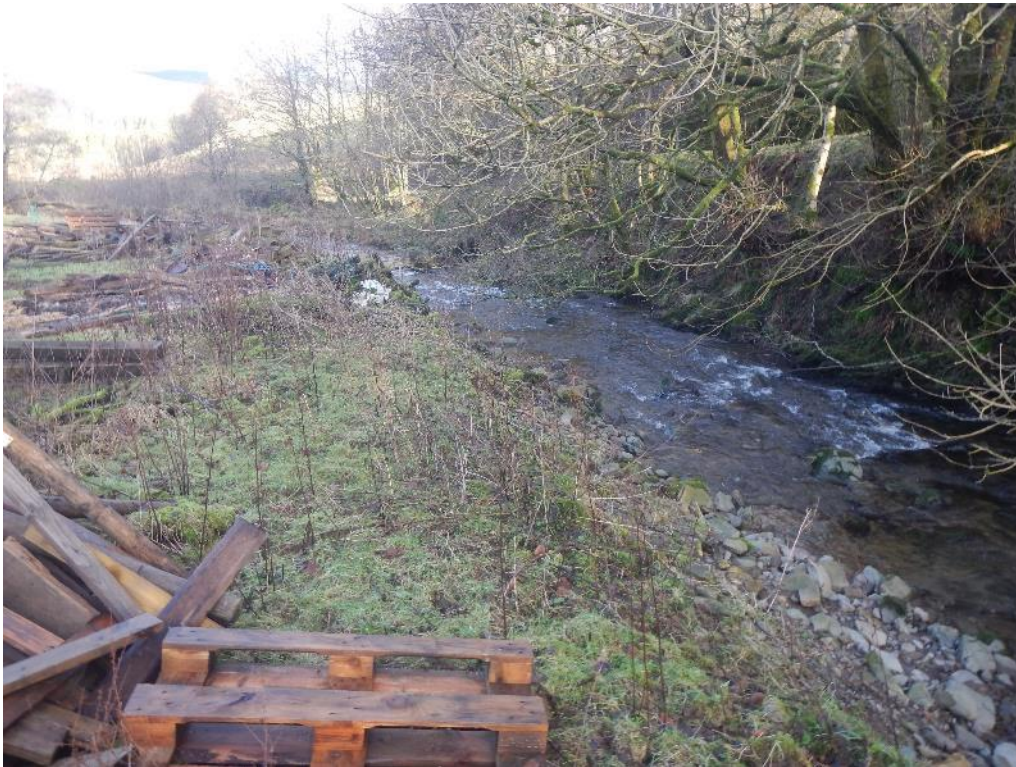
Figure 42. Just d/s of the Glenbertle Burn, the LB of Boyken Burn was being used to store wood and rubbish, with some of the rubbish items sufficiently close to be washed into the burn on a moderately high flow (55.1863, -3.076835).
