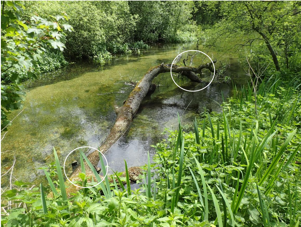
Figure 50. Woody material securely pinned in place with sturdy stakes. The benefit of this technique is that it can be used without nearby trees as an anchor point. Posts (white ellipses) are driven into the bed and/or bank to secure the material, with the butt ends u/s, as material would usually come to rest. Utilisation of this technique is usually in more sheltered inside bends, where it can be incredibly effective at increasing sediment deposition to reshape an over-capacity channel.
