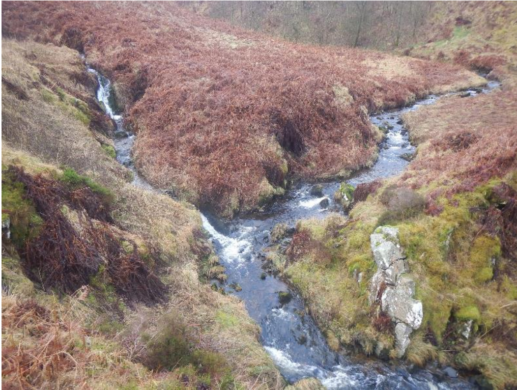
Figure 17. Looking u/s at the confluence with Boyken Burn: even the first 20m create an obstacle to fish (55.1837557, -3.1257363), owing to exposed bedrock (left of shot).
