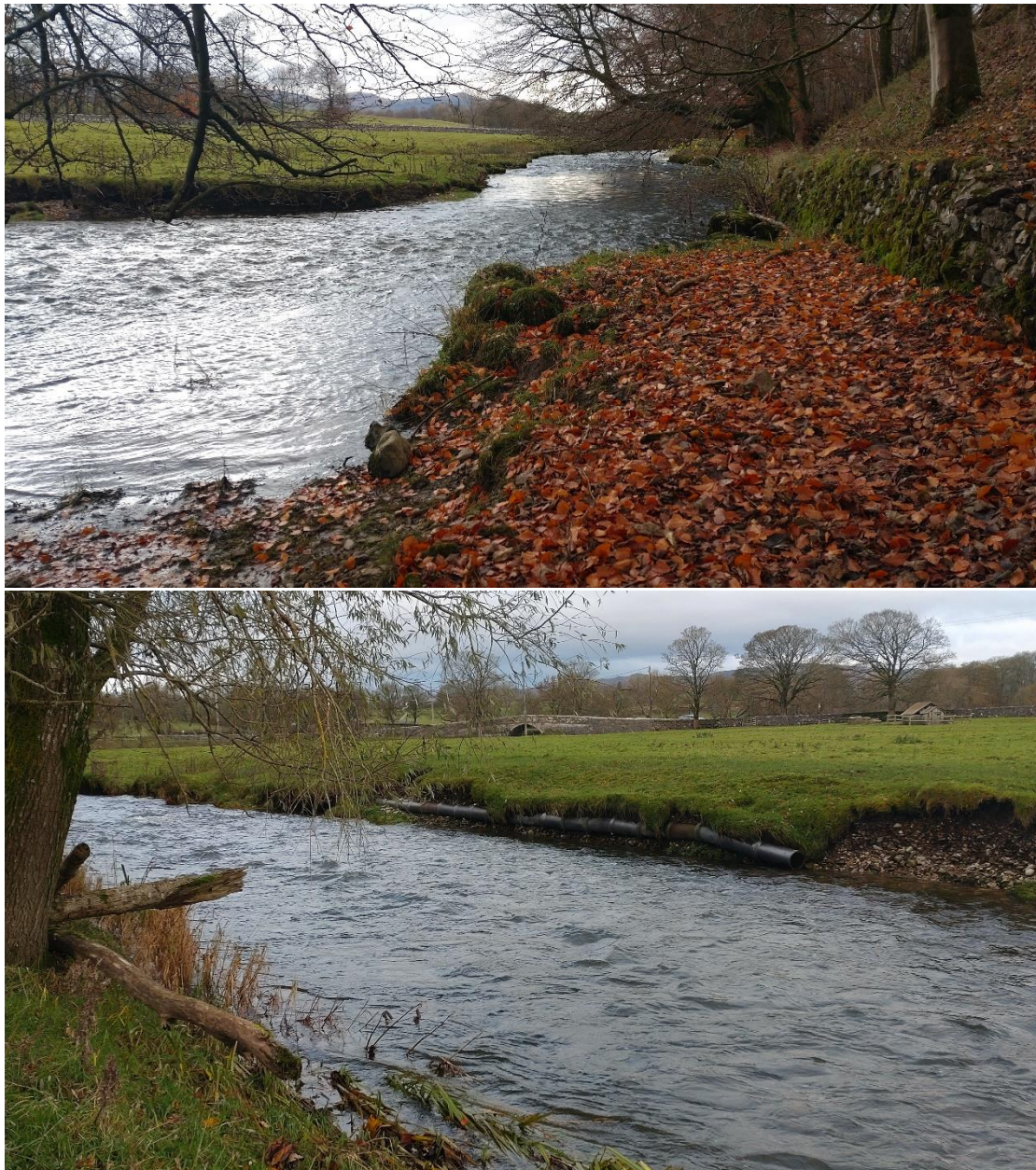
Fig 8. Constraints on the channel. Upper – walling to the RB to accommodate the Pennine Way, and lower – pipework from the pumphouse infrastructure (just visible top right) buried in former alluvial substrate within the LB and now eroding into the channel.
