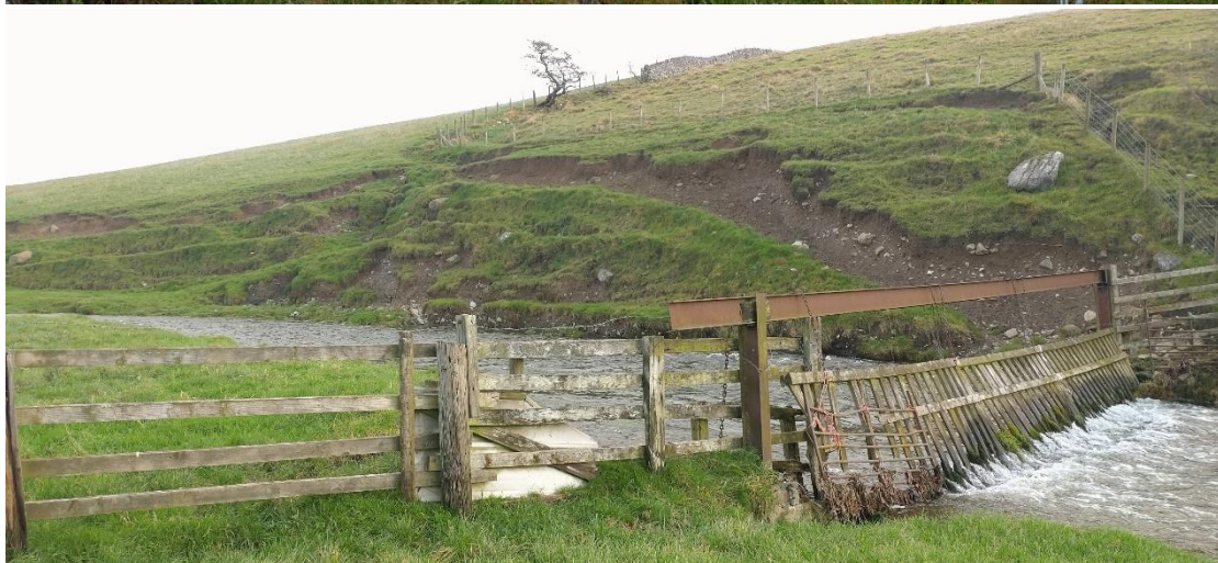
Fig 3. Looking back d/s along a straightened section forced diagonally across the floodplain: overly wide and very exposed. Stock access both banks during low flows. The white arrow identifies the area highlighted in the lower panel where livestock had eroded the hillslope into terraces and bare earth.
