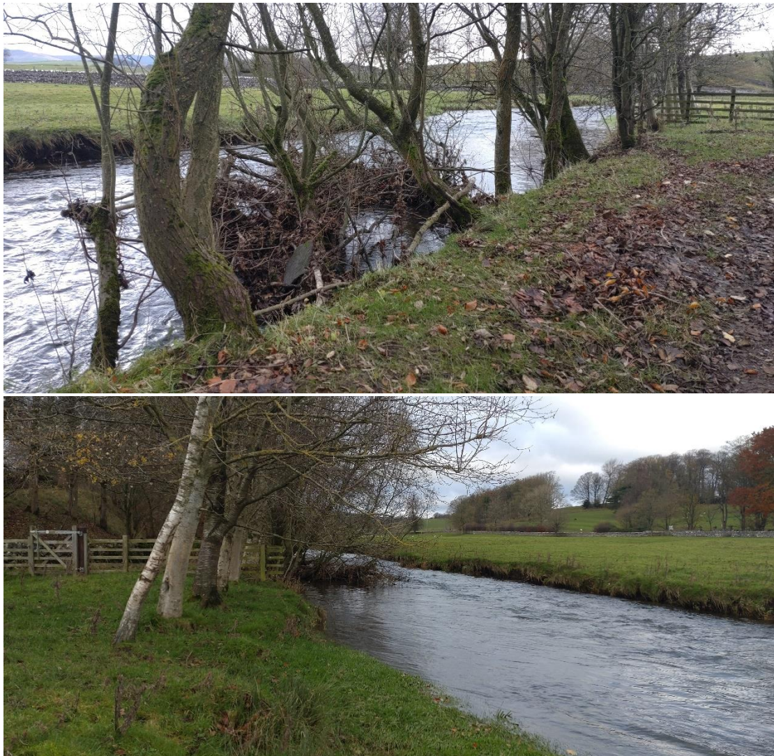
Fig 7. Upper - fine debris trapped in the trailing and submerged stems of willow and alder. When viewed from d/s (lower), the slack water refuge was clear to see. Note the clear browse line on the trees in the field exposed to livestock (lower panel).
