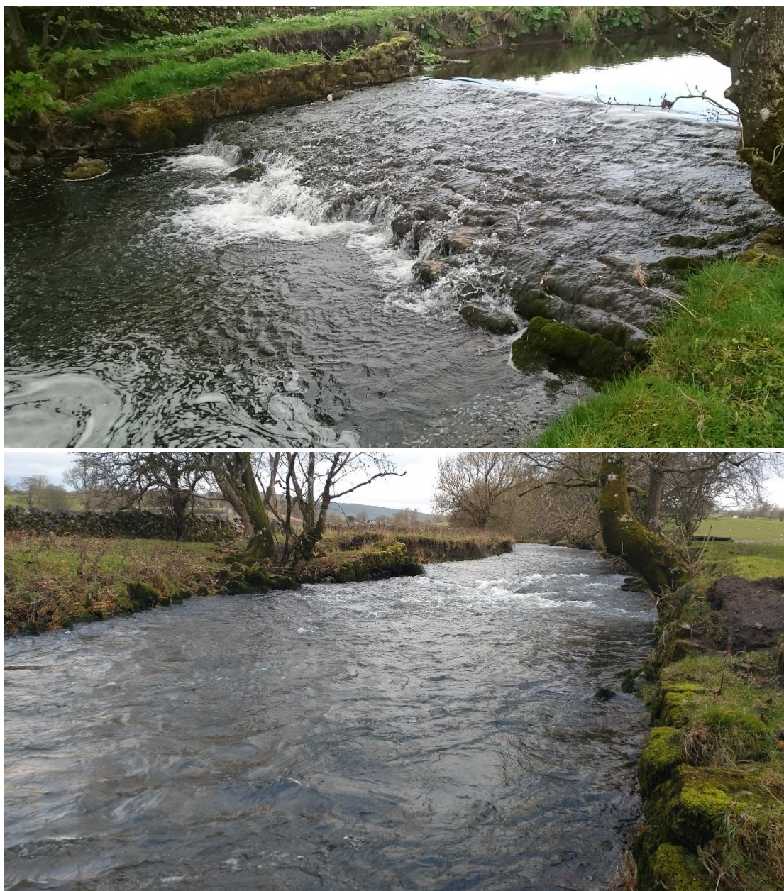
Fig 11. Newfield weir prior to removal in 2021, and the retained wall stubs still visible in 2023 – no longer a barrier to fish or sediment.
