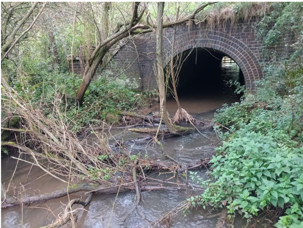
Figure 2. (53.32262, -0.1517844) The culvert beneath the disused railway line has a natural bed gradient and does not present any barrier to the free movement of aquatic organisms nor sediment transport. Woody material within the river channel provides good in-stream habitat.
