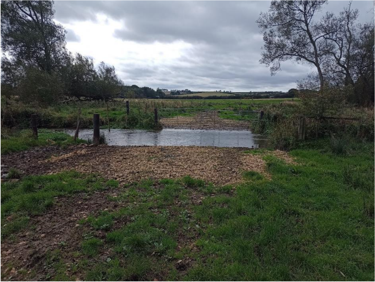
Figure 20. (53.30546, -0.1364610) Ford crossing at downstream end of plantation, just downstream of the Stenigot Beck confluence; view to the west. The use of crushed aggregate is good practice, helping to limit the input of fine sediment to the river.
