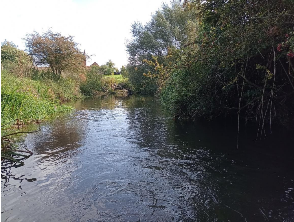
Figure 4 (downstream view; 52.254672, -1.874790). The pool downstream of the footbridge. The meander bend at the downstream end of the pool has been protected with boulder rip-rap. This arrests erosion in the localised area, but can lead to a transfer of energy, shear stress and increased rates of erosion at the boundaries of the reinforcement. Natural approaches to reducing erosion rates are preferable from a river habitat perspective, such as protection with brushwood, establishment of trees on the riverbank and exclusion of livestock.
