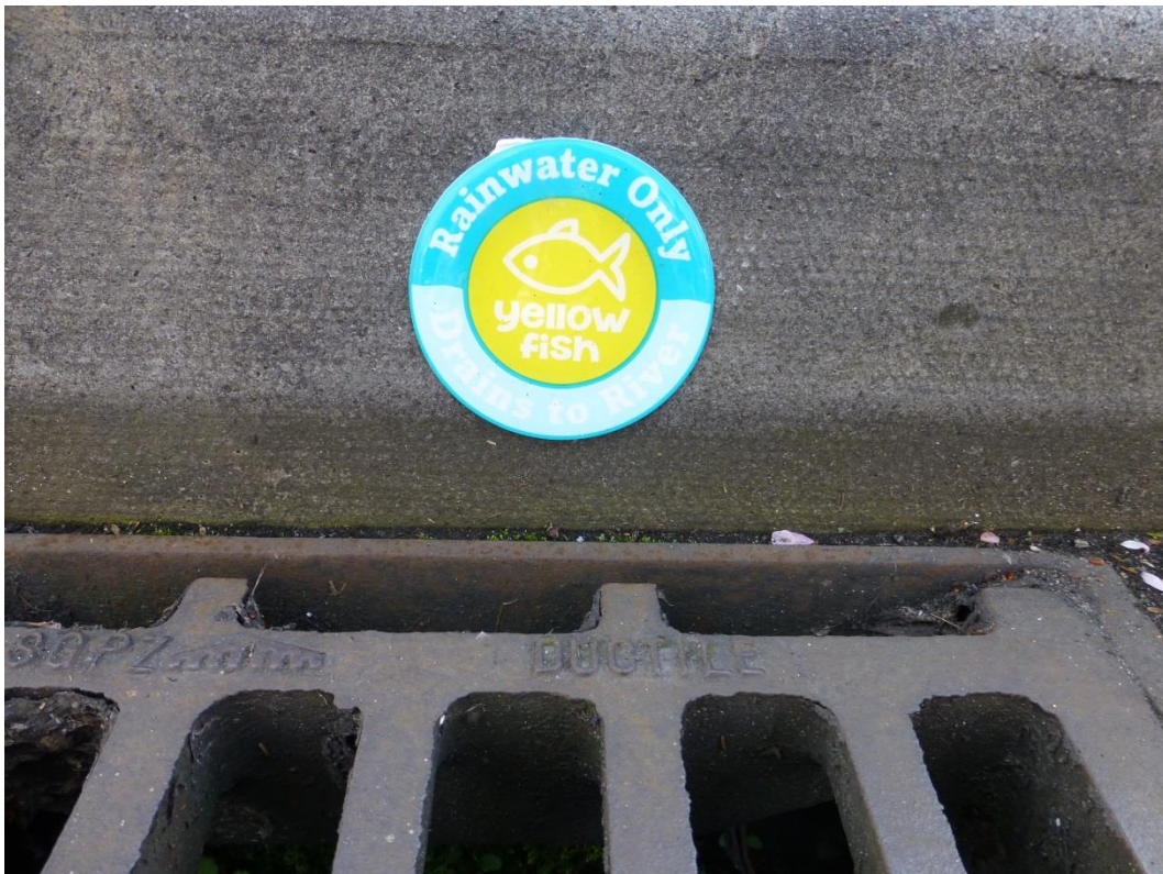
Figure 1 Photo of marker on side of curb next to drain (NB this example would be improved by putting the disc higher up so that the whole back of the disc is directly in contact with the stone.).
