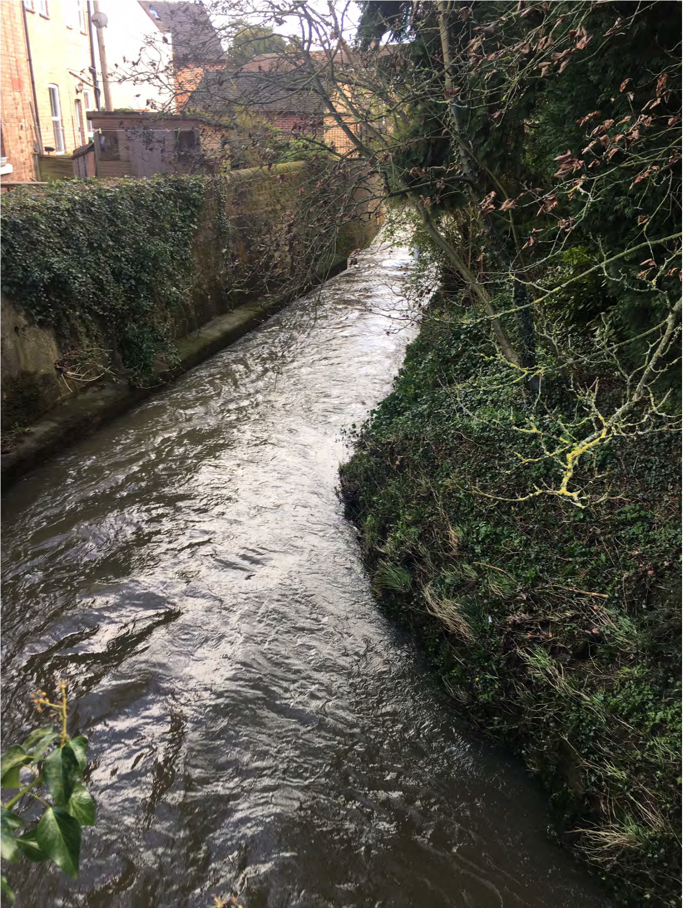
Figure 2.9 Walling lining the river bank
