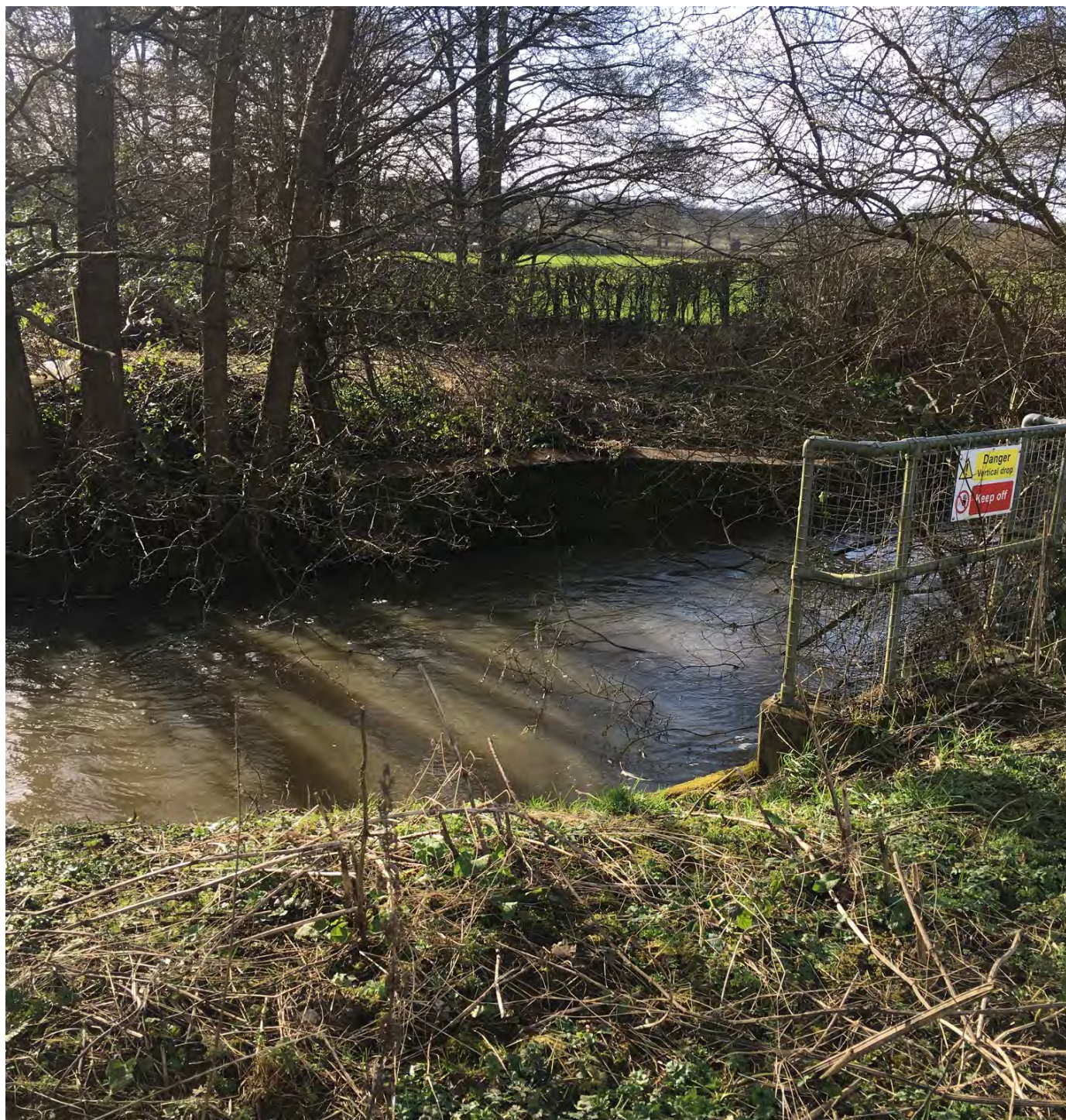
Figure 2.10 Outfall upstream of overspill weir
