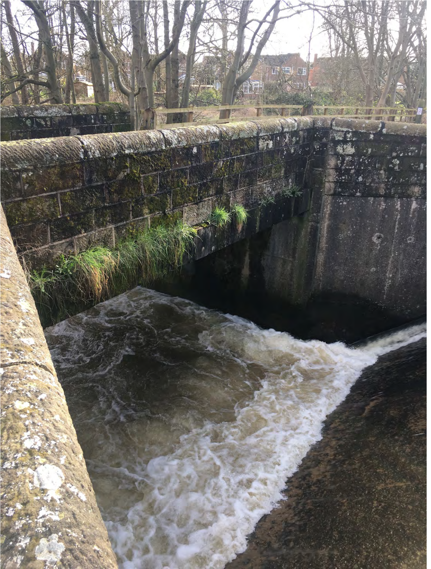
Figure 2.6 Snake Lane weir and access bridge to Duck Island
