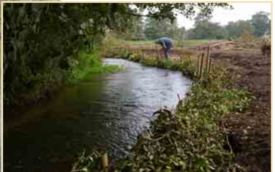
FAGGOT BUNDLES (ABOVE), AND WILLOW SPILING (LEFT), REDUCING EROSION ON THE OUTSIDE OF BENDS.
