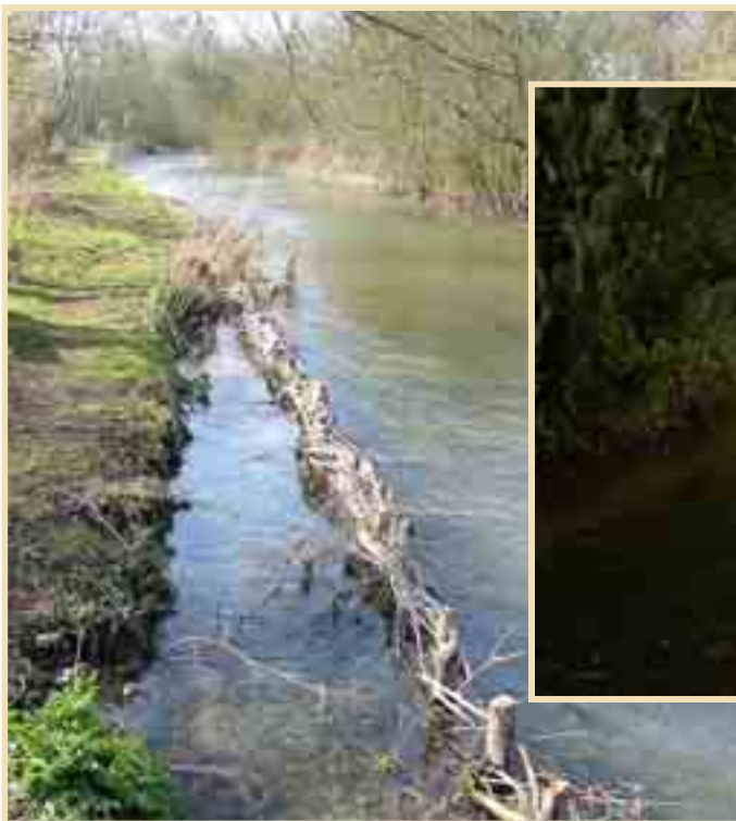
FAGGOT BUNDLES (ABOVE), AND WILLOW SPILING (LEFT), REDUCING EROSION ON THE OUTSIDE OF BENDS.
