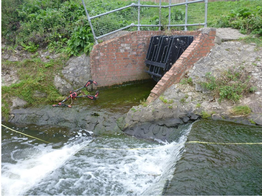
Photo 4 Combined sewer/surface water outfall
