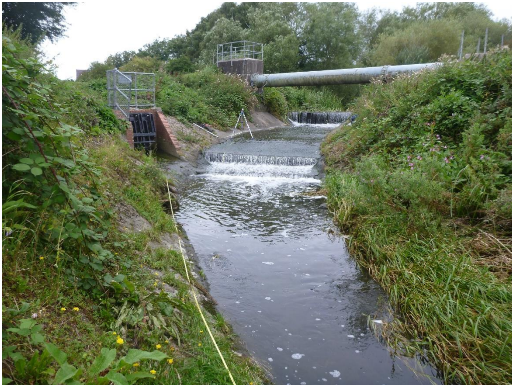
Photo 1 Langley Mill weir
