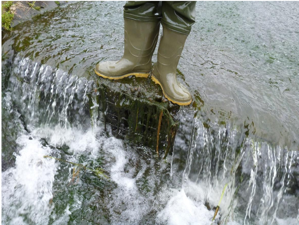
Photo 3 Gabion construction of steps in weir apron.
