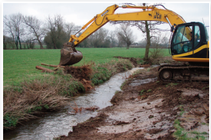
↑ Placing root wads in the channel and re-profiling the banks
