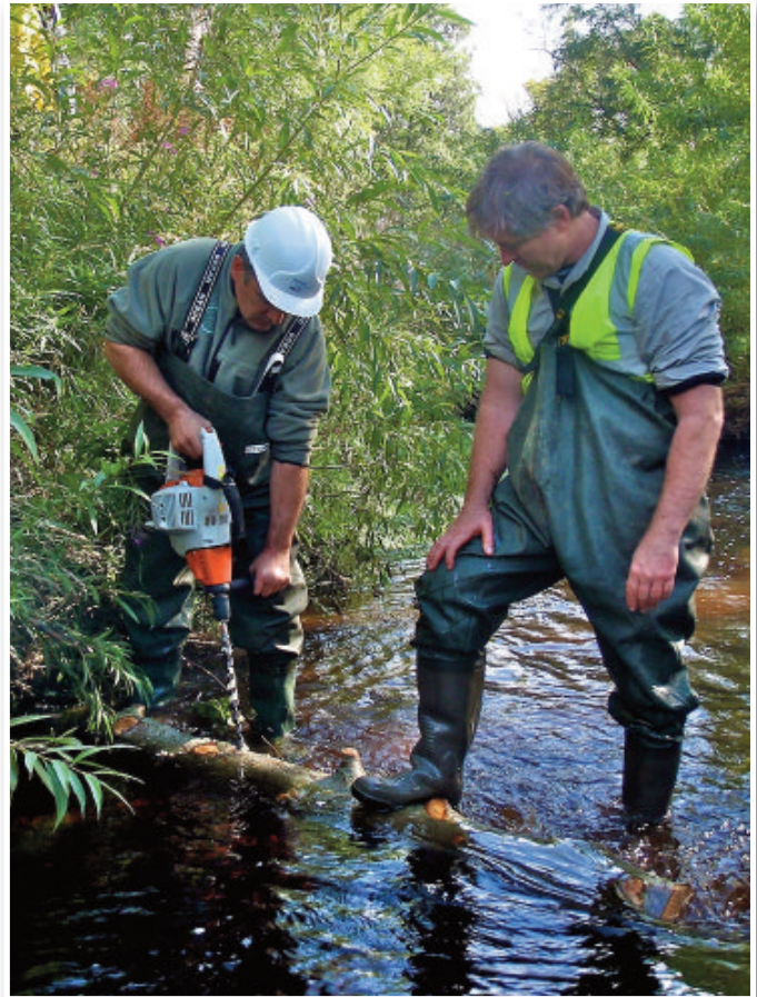
↑ Tim and Shaun installing a flow deflector of the River Peffrey
