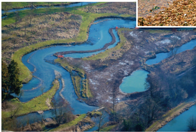
↑ Some of the completed works on the River Kennet
