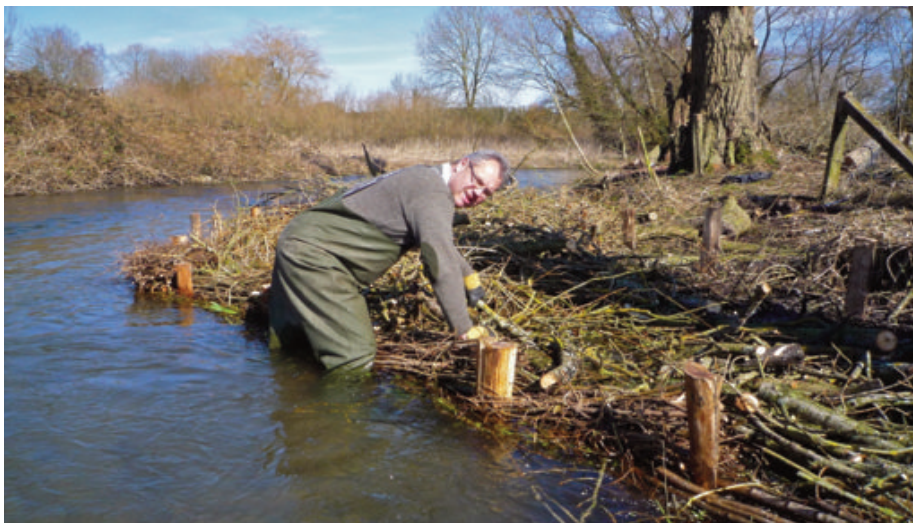
Photo: Volunteer Neil Munday gets to work packing a marginal shelf with brushwood.
