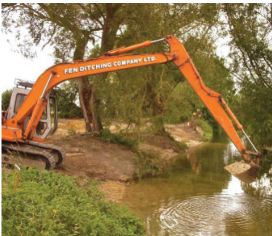
Photo-above: Final gravel placement on the River Cam.
