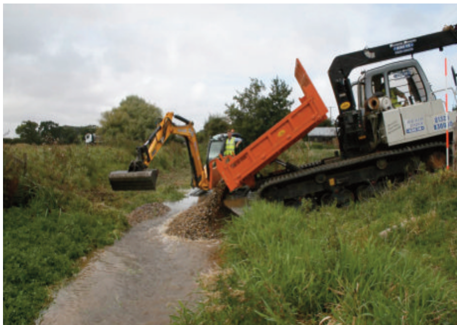
Work on the River Stiffkey riffles.
