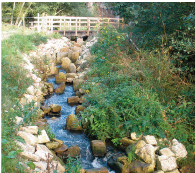
River Hamble – fish pass in operation
