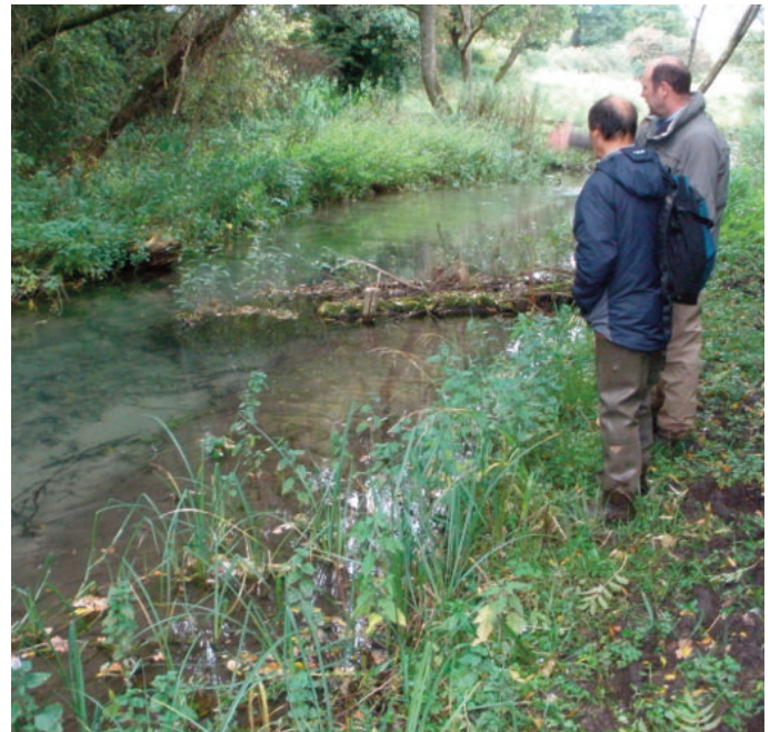
Large Woody Debris Flow Deflector
