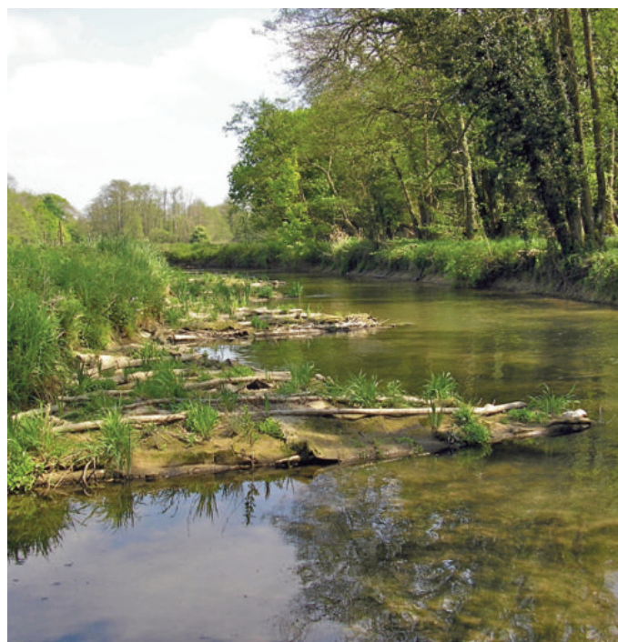
'Dragons teeth' flow deflectors on the R.Nadder
